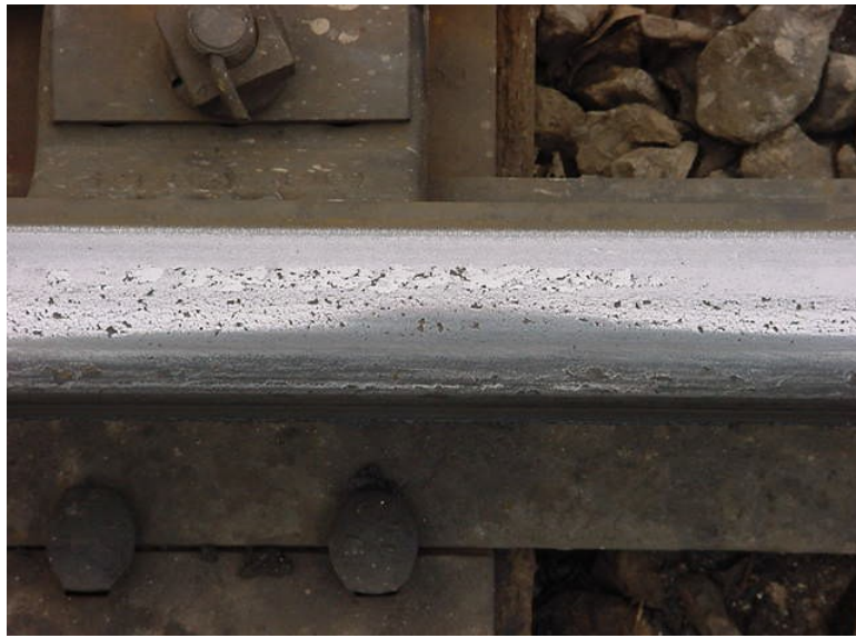
Figure 3-10: Rail Head Checking
