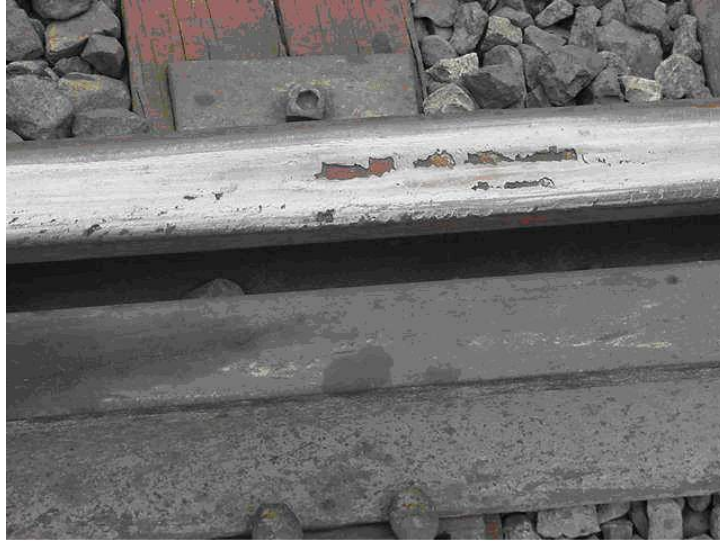
Figure 3-12: Rail Surface Spalling
