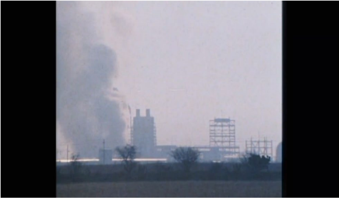
Figure 4-5. Deep Shot of the Tula Electrical Plant. Etnocidio, notas sobre el Mezquital (Paul Leduc, 1977).
