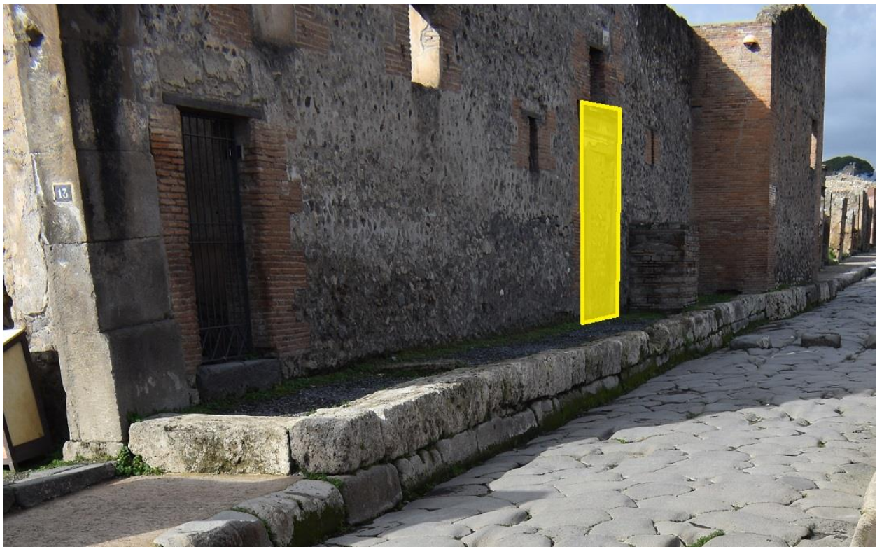
Figure 40 - Image of the Stabian Baths addition that completely blocks western sidewalk seen in the upper right portion of the image, and curbstone elevation achieved with an additional row of pavers. Entrance blocked in antiquity highlighted.
