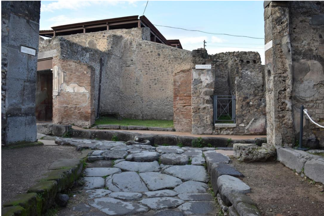
Figure 16 - Photo of Intersection B, looking north along Vicolo del Lupanare. Large ramp in the foreground prevents vehicular traffic from entering Vicolo del Lupanare from Via degli Augustali.
