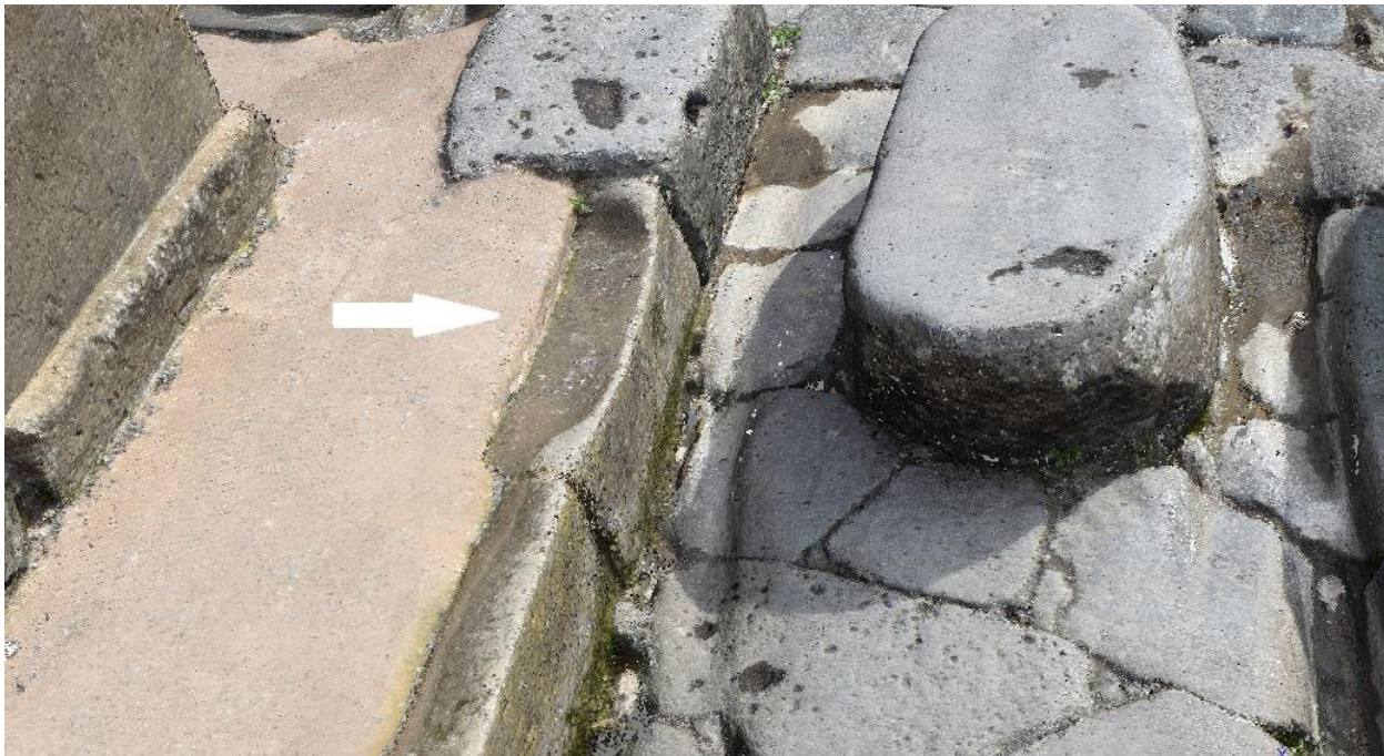
Figure 41 - Image-based model of detail of curbstone in the northern branch of wear showing a significant amount of usage, accommodating crossing to the west along the northern side of the stepping-stones.
