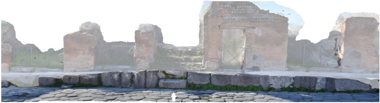
Figure 33 - Section of western side of the northern branch of Intersection A highlighting the increase in elevation as one approaches the intersection with a pair of steps.
