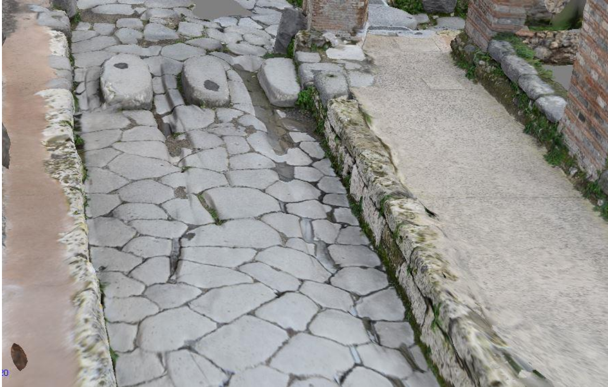
Figure 38 - Photogrammetric model of northern branch of intersection C. Notice the two height curbstones and the difference in sidewalk width between the eastern and western sides. The western sidewalk easily accommodates two-way traffic, while the eastern branch is more suited for one-way traffic.
