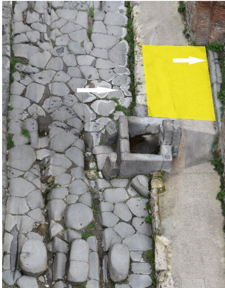
Figure 39 - Photogrammetric model of the southern branch of Intersection C. Highlighted area is the extra space created by the bending outward of the curbstones and the westerly shift of the facade (indicated by the arrows).
