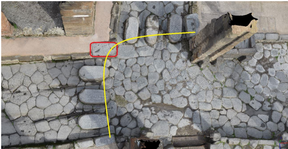
Figure 42 - Image-based aerial of model with preferred path of travel highlighted in yellow and transition stepping-stone in red. Also, notice the angling of the hybrid curbstone/stepping-stone that is directly behind the water tower. This angling encourages people to move away from the water fountain as they enter the southern sidewalk.
