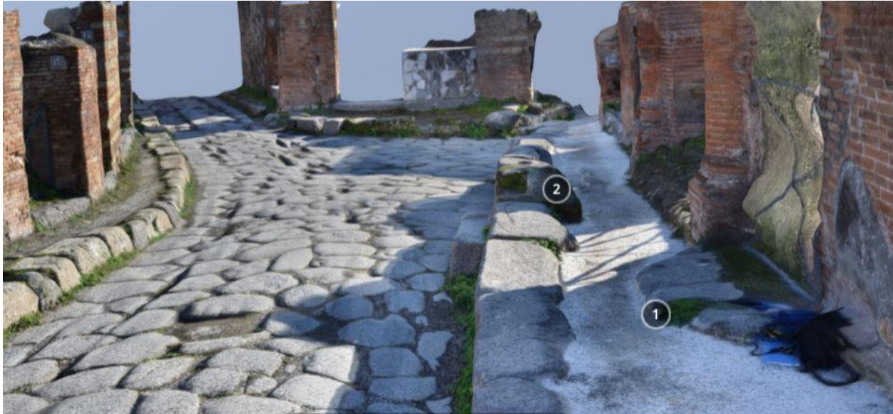
Figure 34 - Image-based model of Intersection A: 1) Bottleneck caused by protrusion of threshold 2) Bottleneck caused by upper step narrowing sidewalk.
