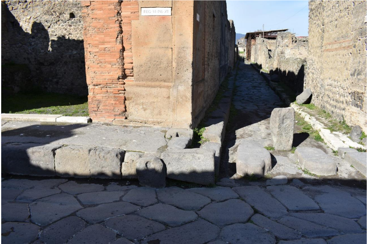
Figure 23 - Photo of Intersection E, looking north. The later blocking stone to prevent vehicular traffic from entering Vicolo del Labirinto can be seen in the center left of the image.
