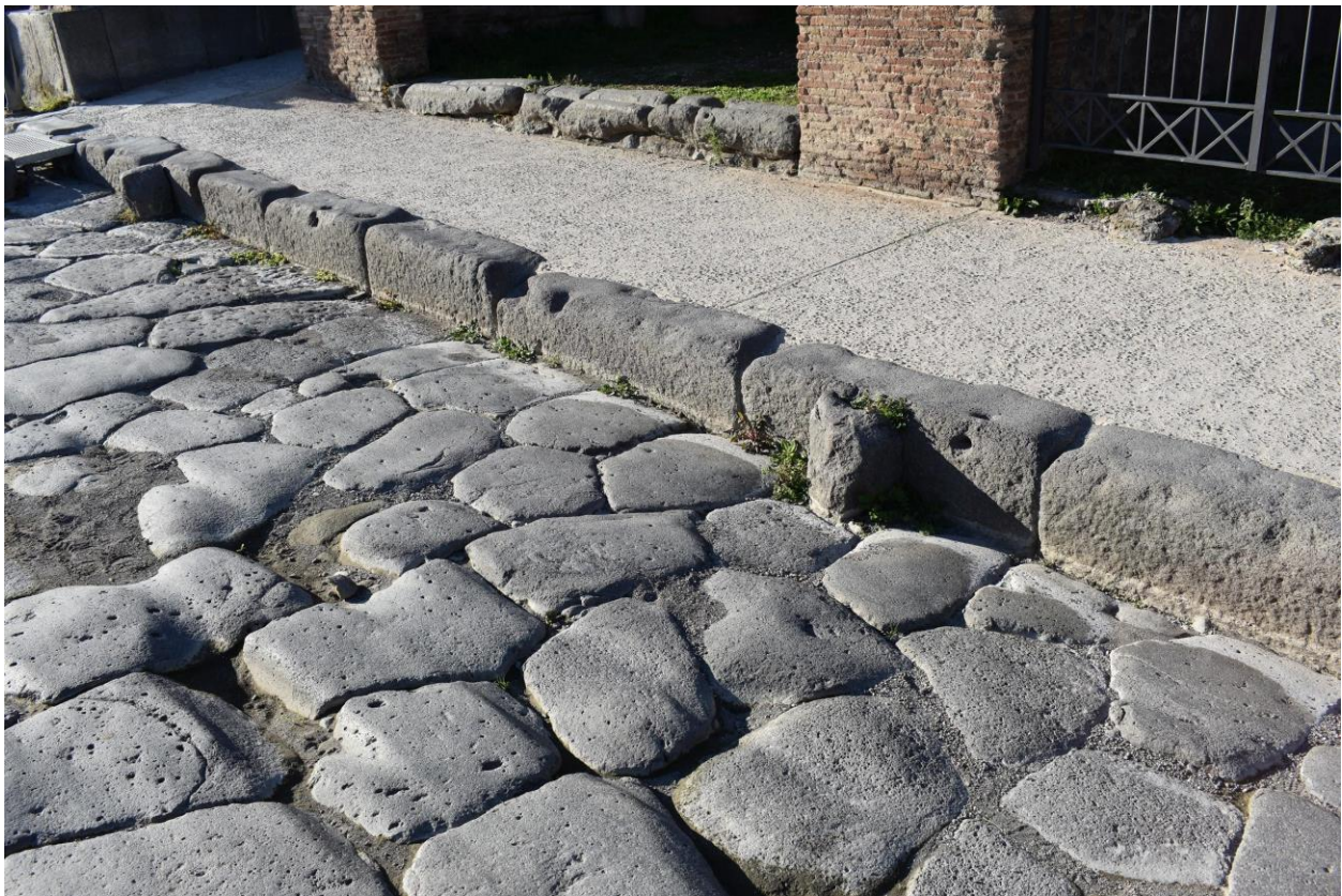
Figure 26 - Photo of western branch of Intersection F showing a pair of hitching holes and narrowing stones.
