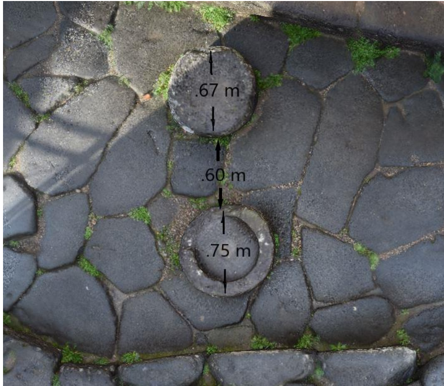
Figure 9 - Image-based model of Intersection C showing the smaller width of the two stepping-stones in the middle of Intersection C. Just a small width would not suffice for two-way crossing. The space between them is also wider than a comfortable crossing length.
