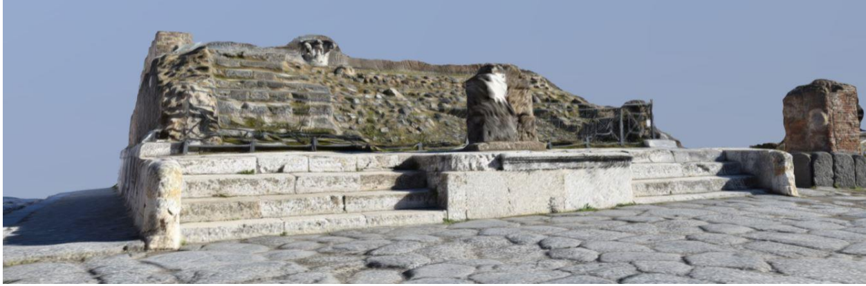
Figure 48 - Image-based model of the steps leading to the Temple of Fortuna Augusta that functioned as places for pedestrians to rest adjacent to the large vehicular free zone in the southern branch of intersection G.
