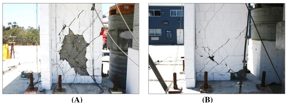
FIGURE 9 Damage in Specimen 1 after MUL-133%: A, south view of Wall 1; B, north view of Wall 2
