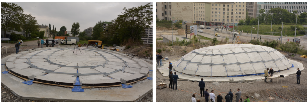
Figure 2.25: Pneumatic wedge system. Adapted from [100]
