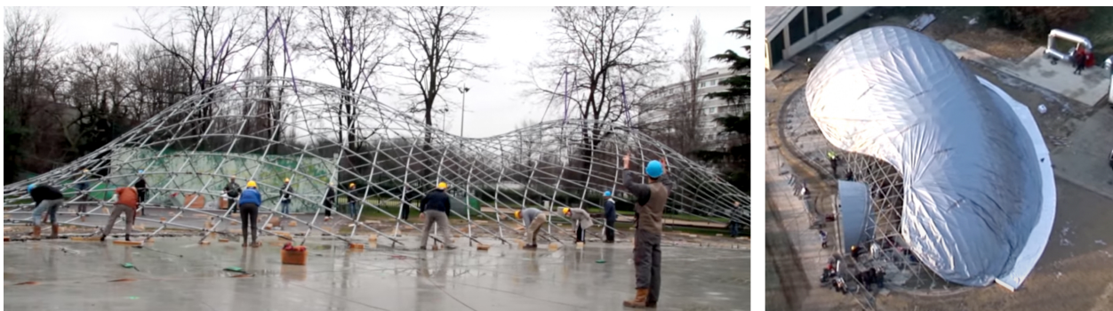
Figure 2.10: The Ephemeral Cathedral of Créteil (Paris, France), a gridshell structure made of composite materials, 2013 [38].
