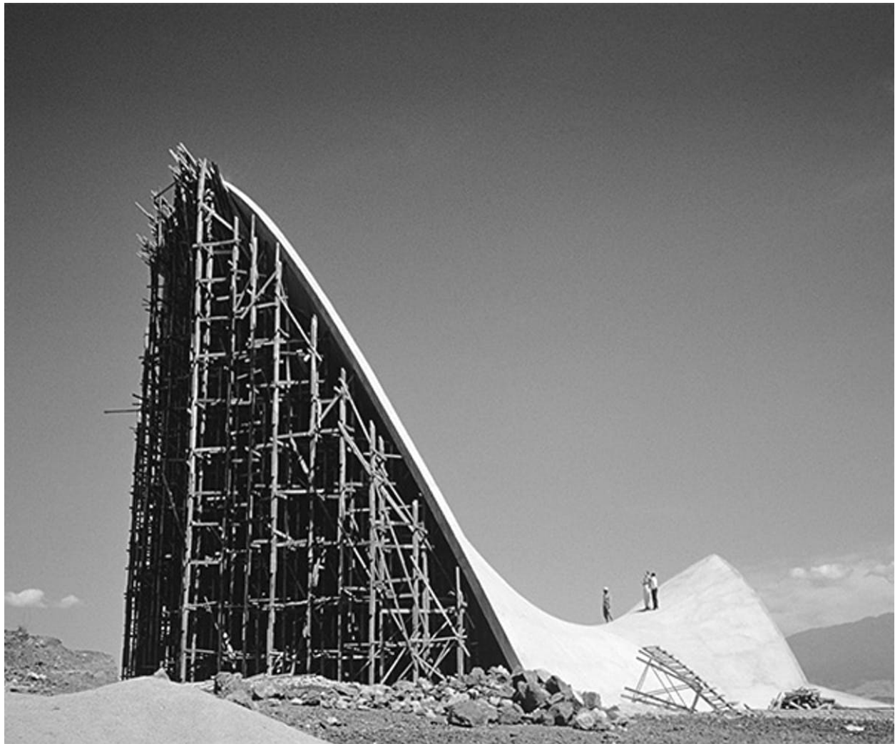
Figure 2.17: Highly complex and intensive labor casting process of Felix Candela's shells in Mexico. Adapted from [66]
