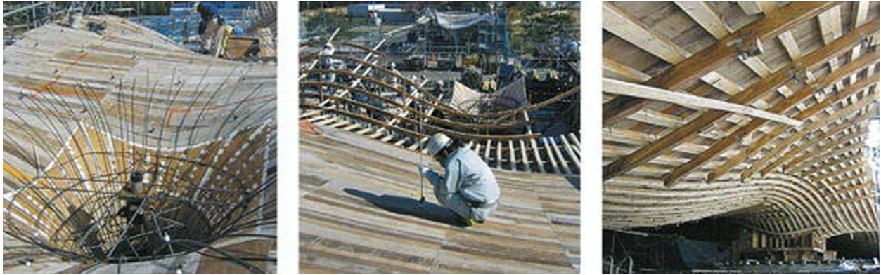
Figure 2.18: 'Meiso no Mori' Municipal Funeral Hall, Kakamigahara Japan. Concrete roof. Adapted from [70]
