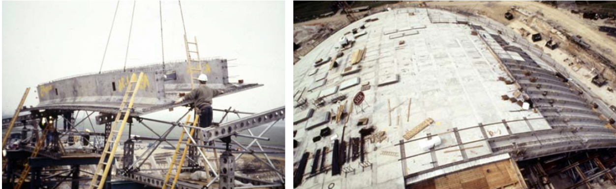
Figure 2.21: Nine hundred precast concrete panels are hoisted into position before concrete is poured onto the top surface to stitch the panels together. Adapted from [71]
