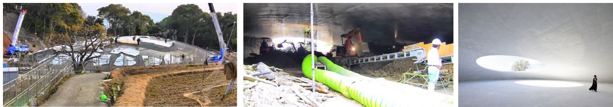
Figure 2.23: Teshima Art Museum: Earth mound as formwork. Adapted from [82]
