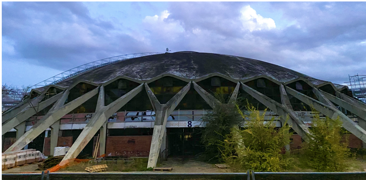
Figure 2.4: Palazzetto Dello Sport (1960) by Pier Luigi Nervi, Rome. Photograph taken by the author, Yasaman Yavaribajestani.
