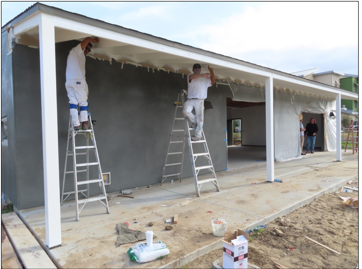
Workers putting some of the finishing touches on the "gator barn".
