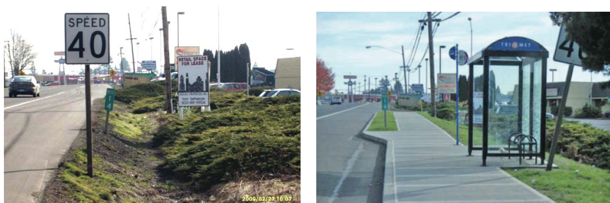
Figure 6.13: SW Oak & 17th – Before and After Line 57-TV Highway Improvements Source: Young Park, TriMet
