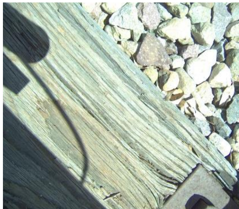
Figure 6.11 Typical image showing tie and ballast captured by the camera
