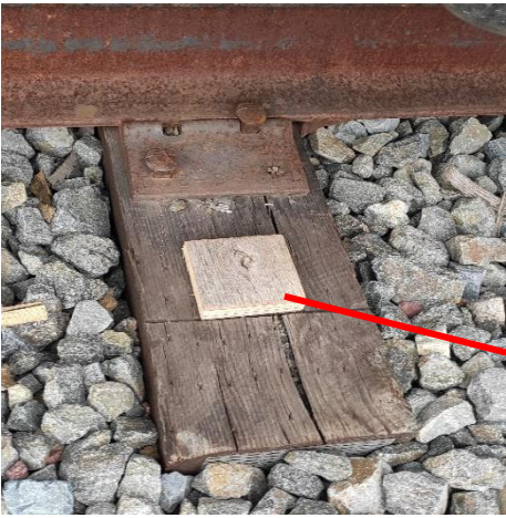
Figure 7.9 Wood block placed on one of the ties
