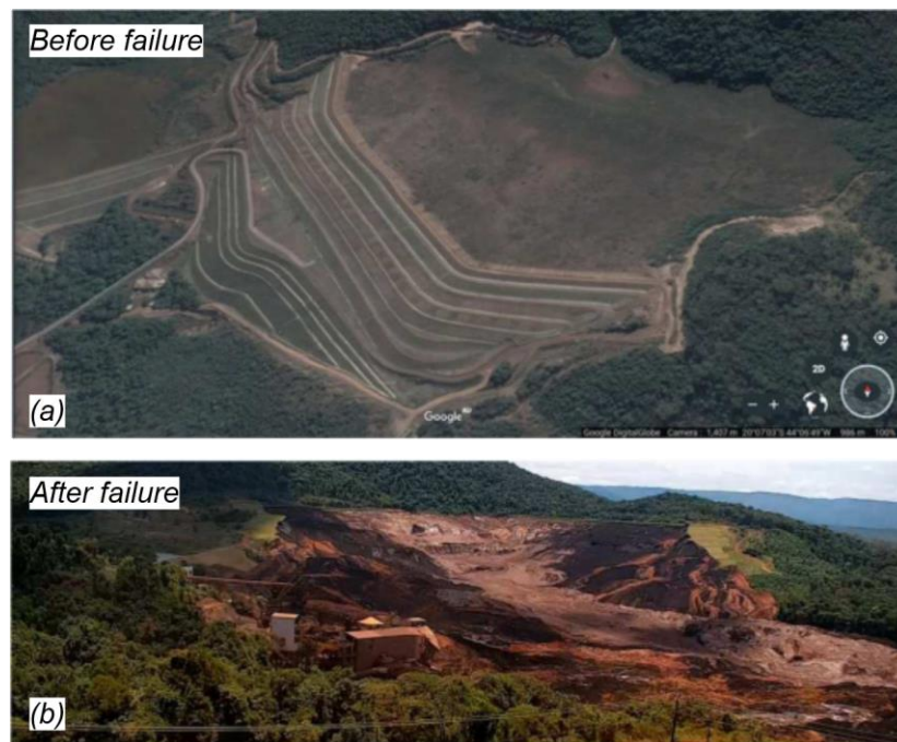
Figure 4-1: Feijão Dam 1 (a) looking north prior to failure (Google Earth via Robertson et al. 2019) and (b) after failure (Robertson et al. 2019)
