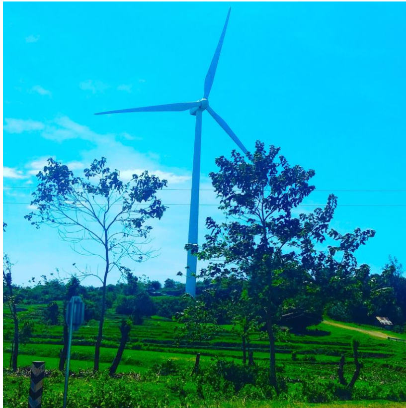
A wind turbine of the San Lorenzo Wind Farm in Guimaras Island, surrounded by verdant rice fields and farmlands. (Photo by the author)
