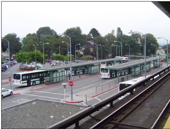
The Bayfair station in Alameda County, California, where AC Transit buses and Bay Area Rapid Transit (BART) trains share a transfer point.
