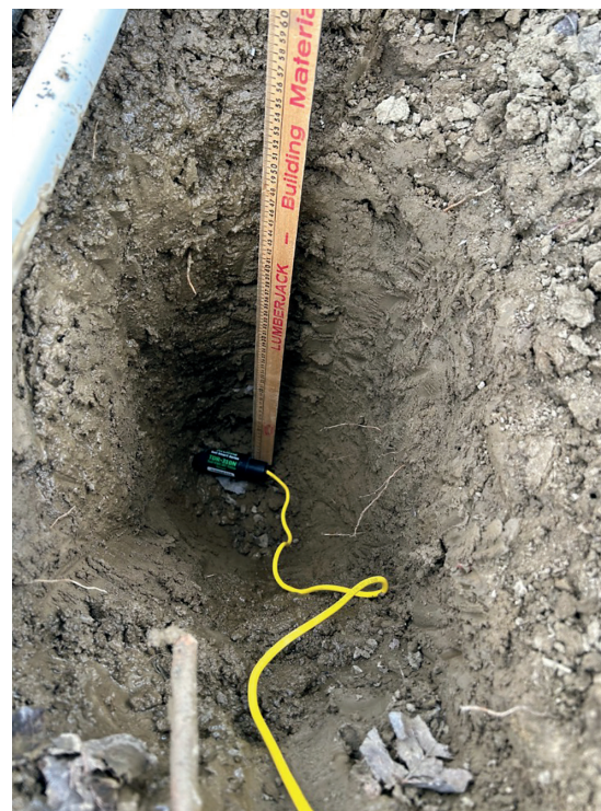
Installing soil moisture sensors at an on-farm pistachio demonstration trial in Fresno County. Photo: Ben Halleck.
