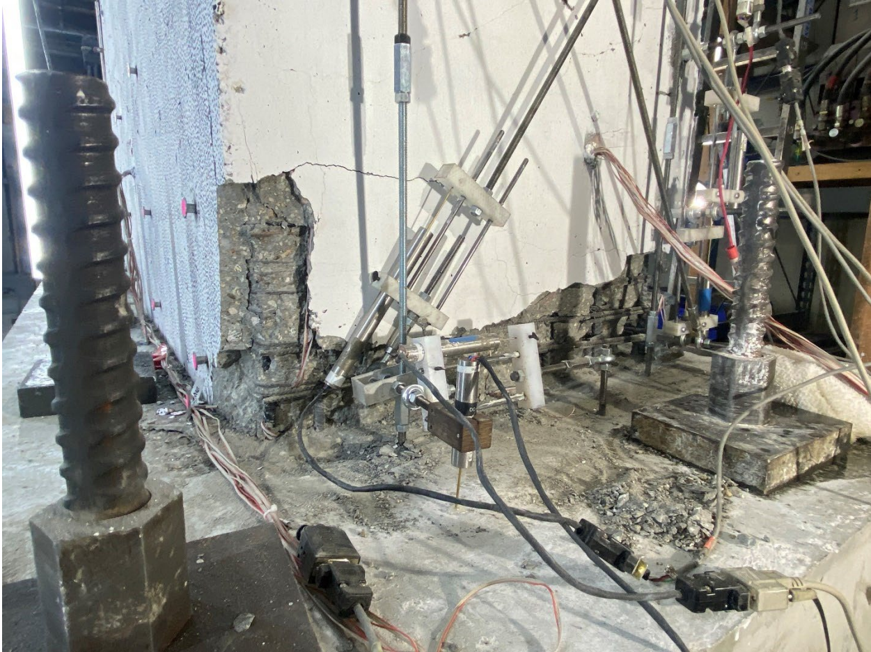
Figure 5-10: East flange after the completion of WLP, CW-2
