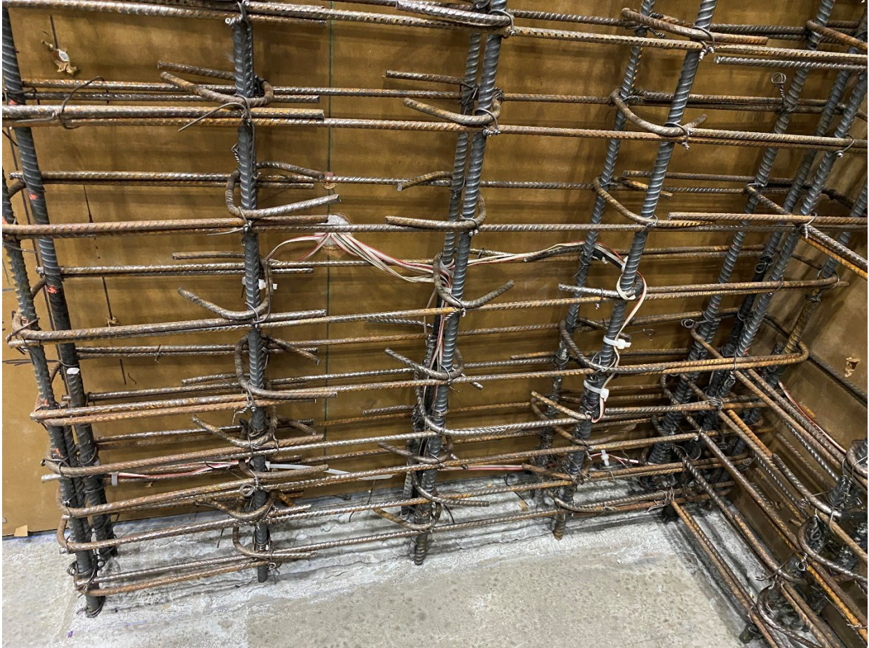
Figure D-5: CW-1 Flange reinforcement close-up
