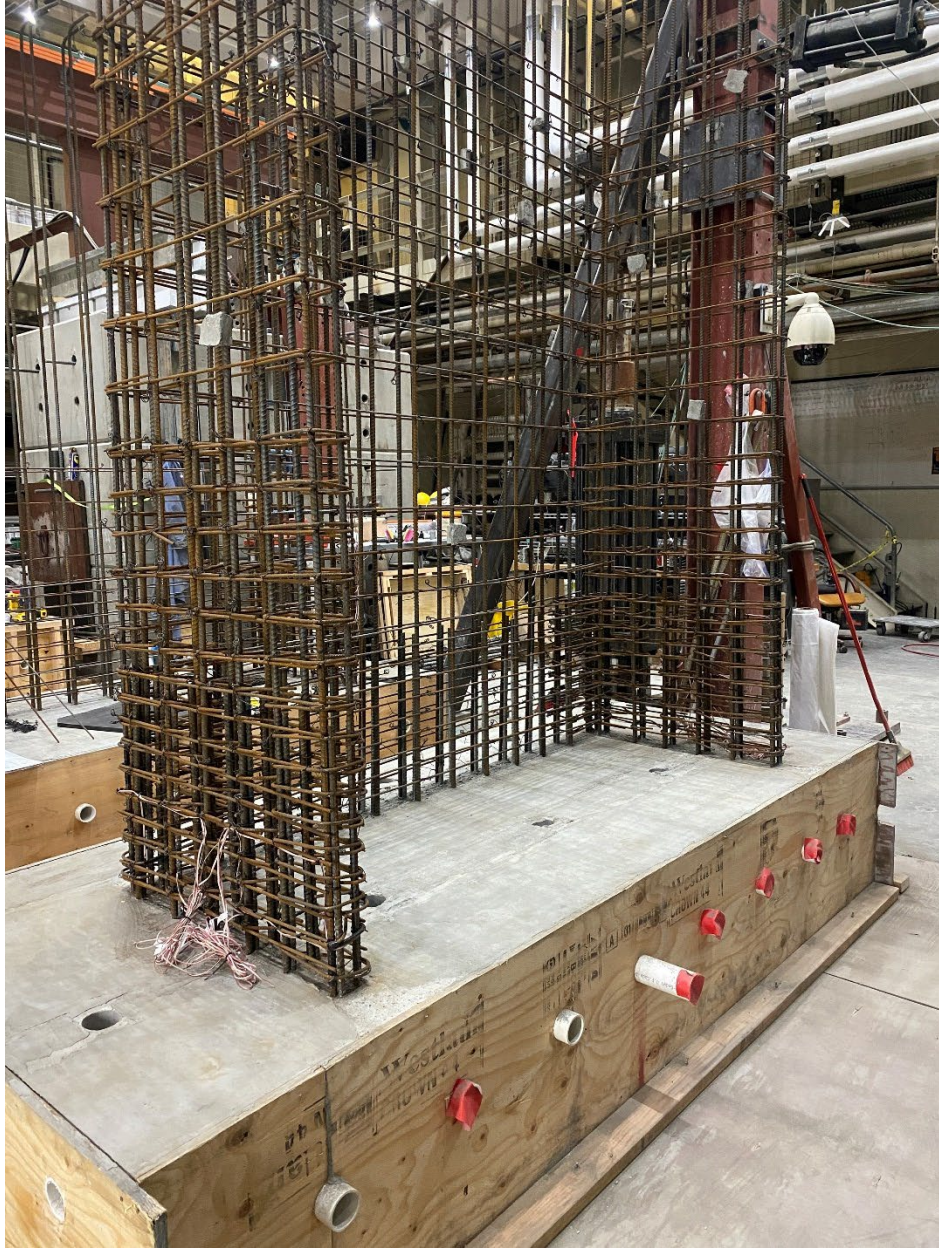
Figure D-10: CW-3 Reinforcement cage
