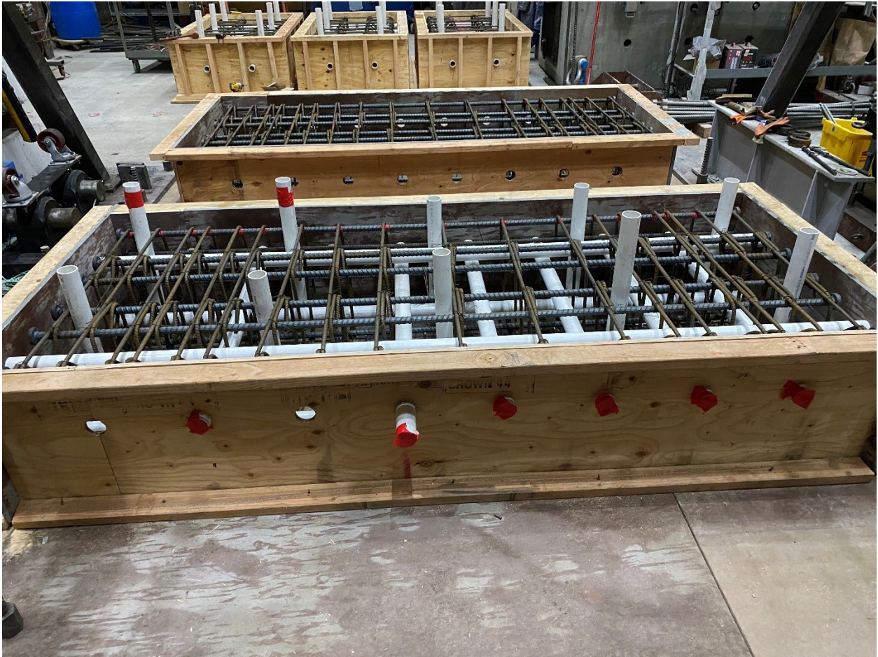
Figure D-9: Phase-II footing formwork and reinforcement cages
