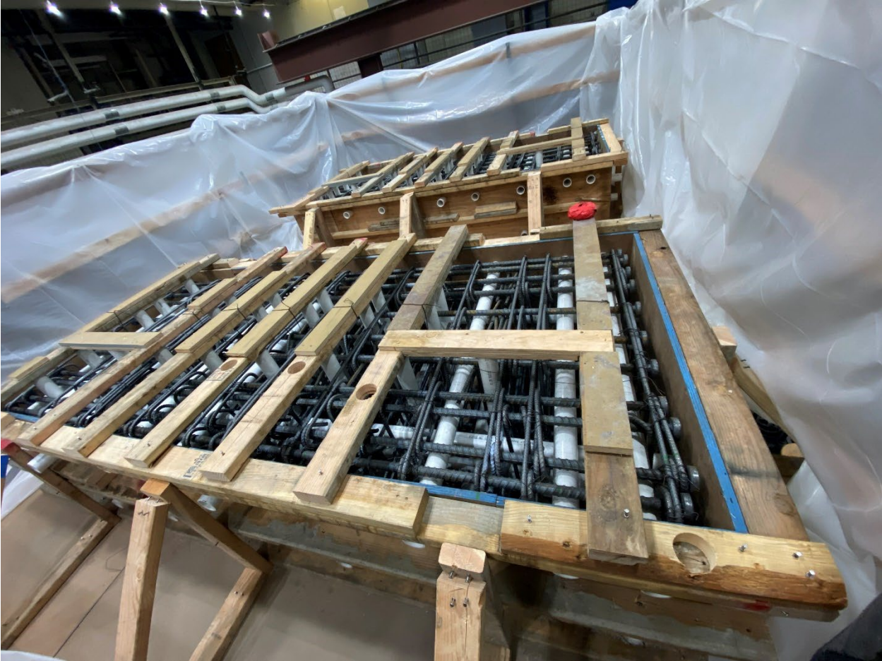
Figure D-8: Top cap formwork and reinforcement cages
