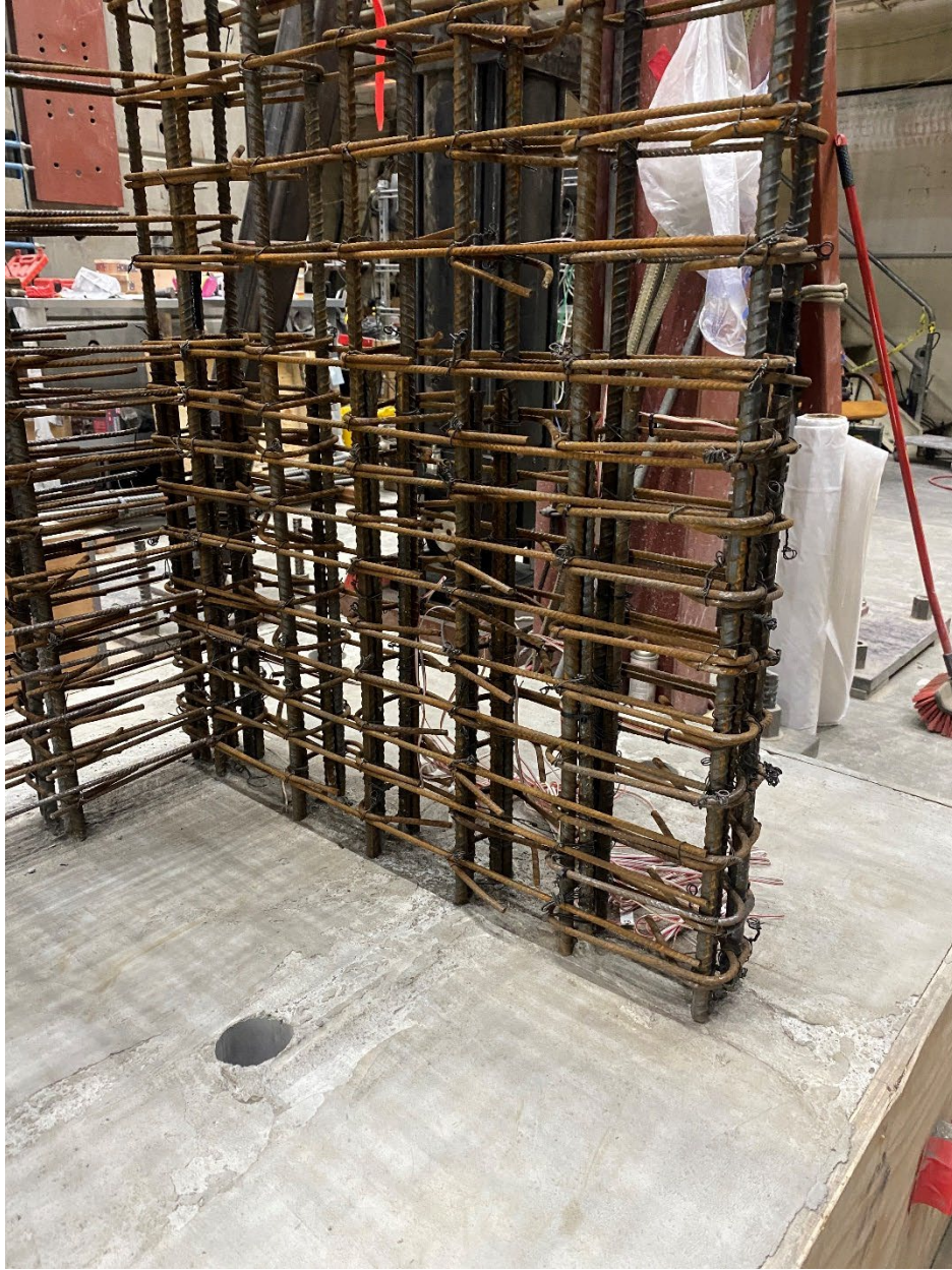
Figure D-11: CW-3 flange reinforcement close-up
