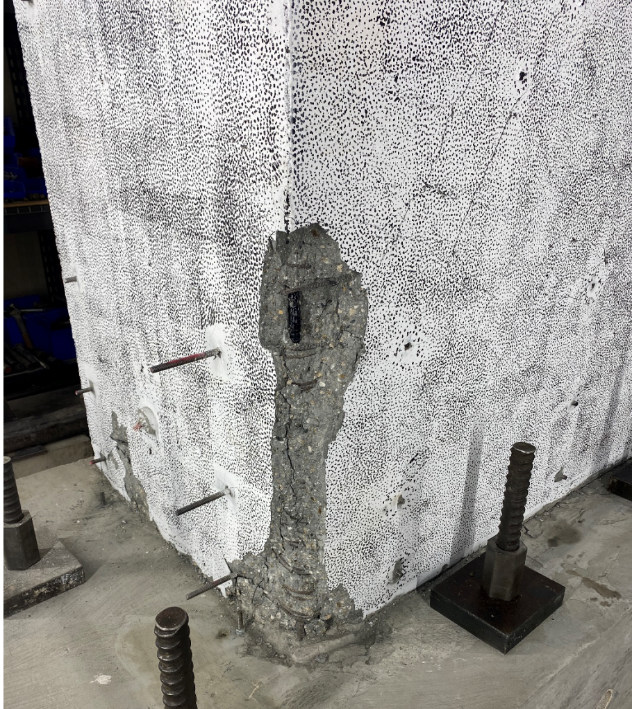
Figure 6-5: Buckling of the west flange corner bar above the spliced region, after three cycles at \pm 1.35\% IP hinge rotation demands, CW-3
