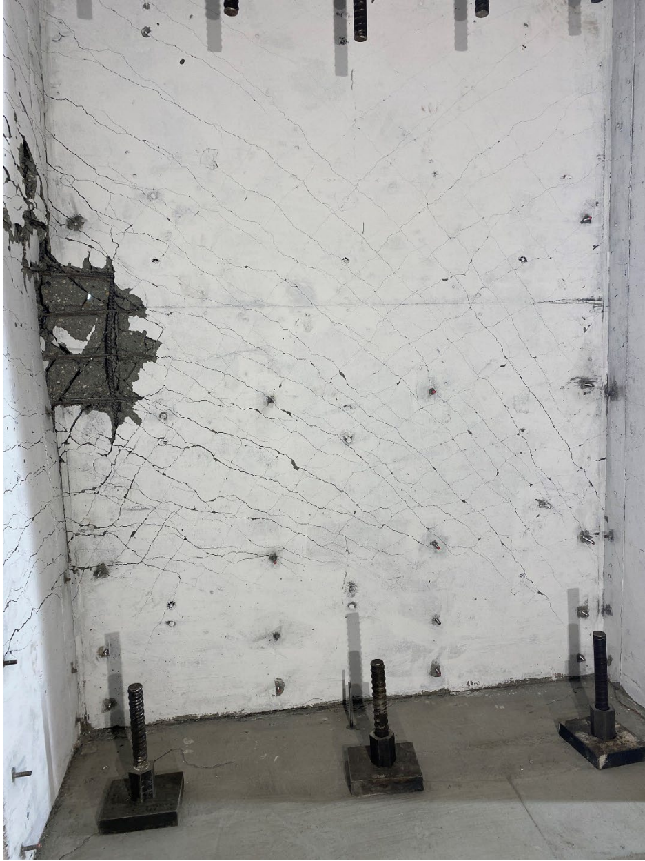
Figure 6-6: Bar buckling and concrete crushing at around 40 in to 52 in. above the footing on the inner surface of the web, after the completion of testing, CW-3
