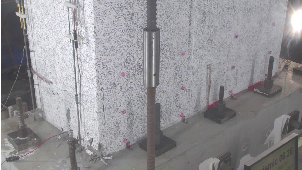
Figure 4-1: Damage state of the West flange and the web after two cycles at 1.5% hinge rotation demands (at zero loads)
