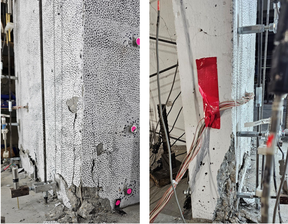
Figure 5-4: West flange corner (left), West flange edge (right) after the ramp-up loading of WLP, CW-2
