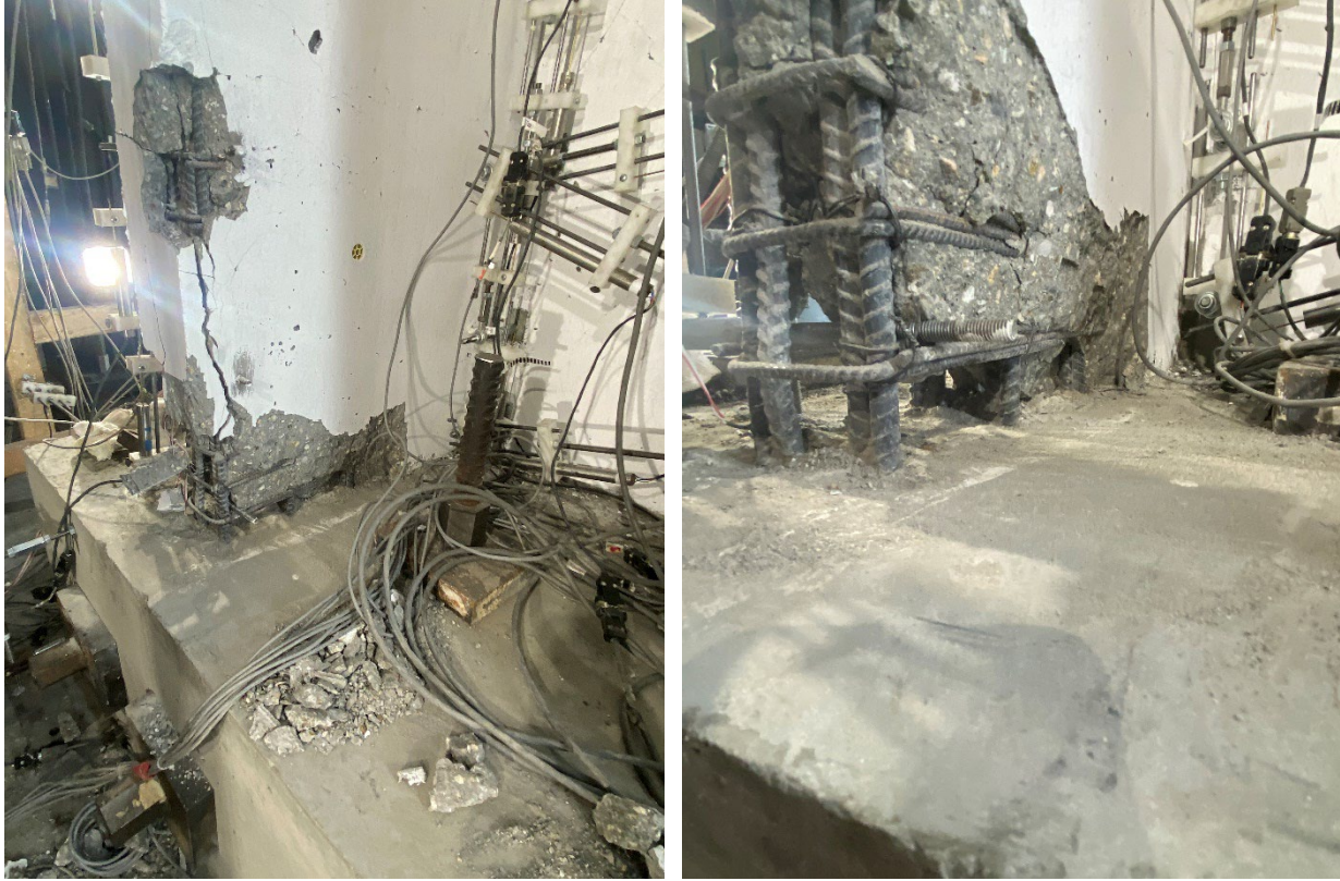
Figure 5-9: East flange edge after the completion of WLP, CW-2
