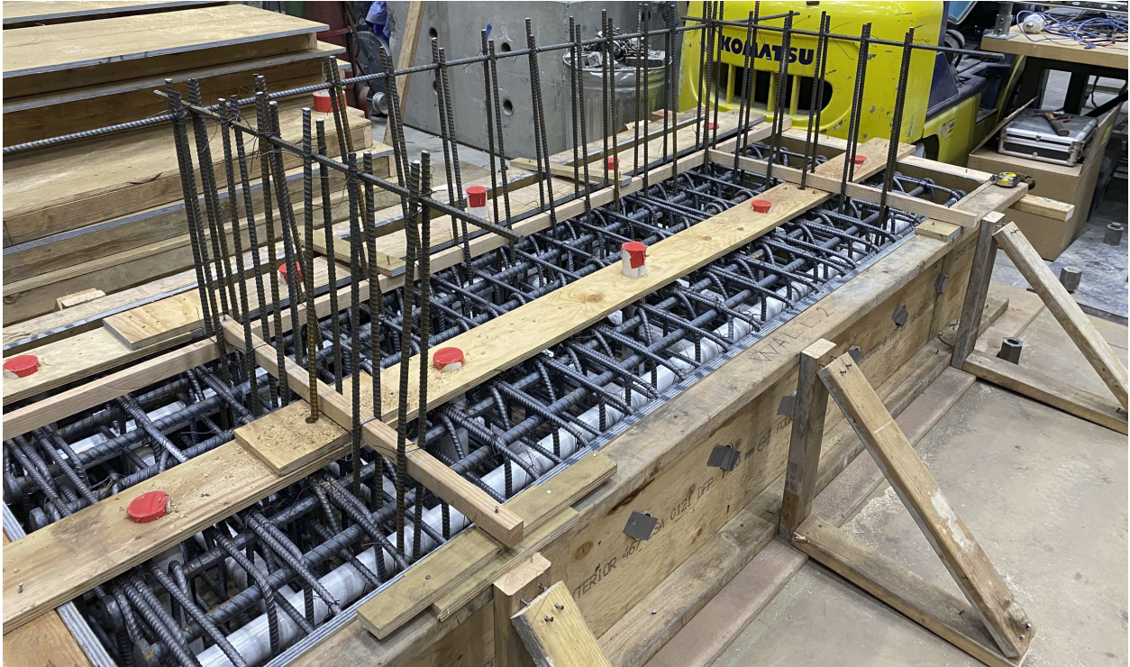
Figure D-2: CW-2 Footing rebar cage with the starter bars
