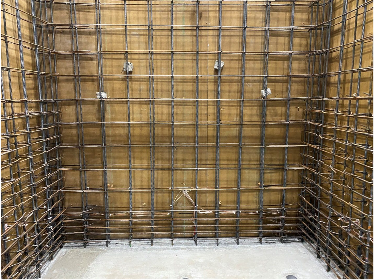
Figure D-3: CW-1 Rebar Cage
