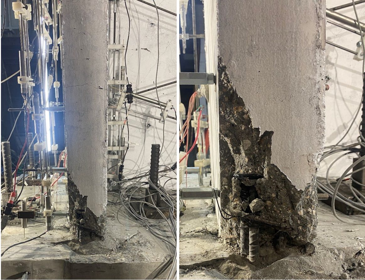
Figure 5-15: East flange edge after the inelastic ramp-down cycles of WLP, CW-4
