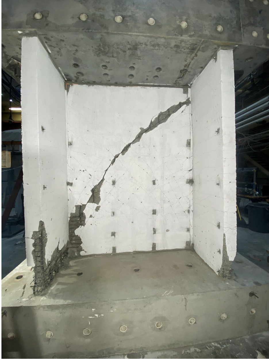
Figure 6-3: Inside surface of the wall after the completion of testing, CW-2
