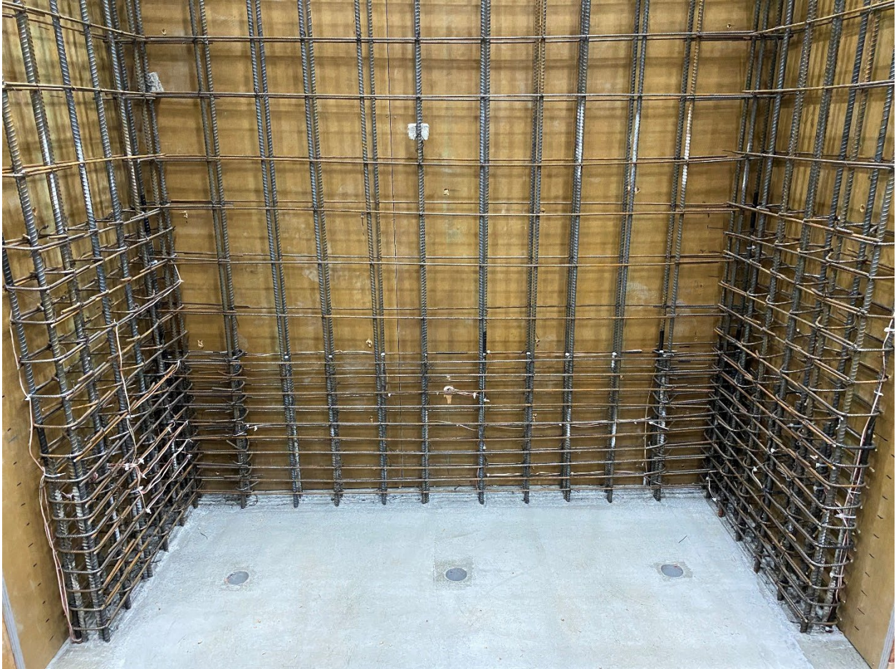
Figure D-6: CW-2 rebar cage
