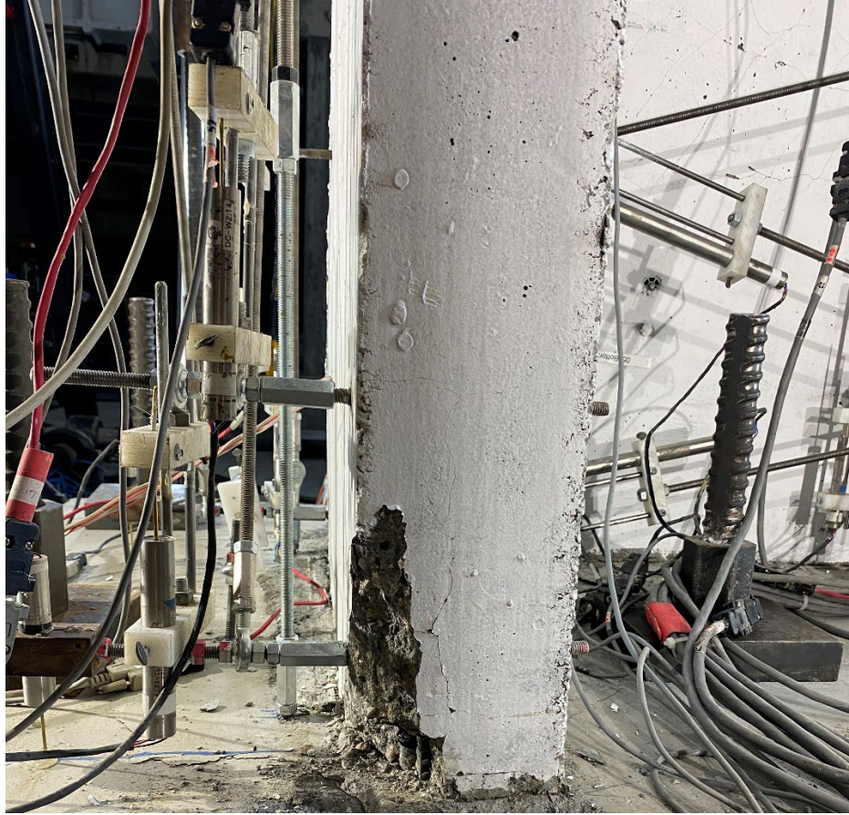
Figure 5-11: East flange edge after the completion of WLP, CW-3
