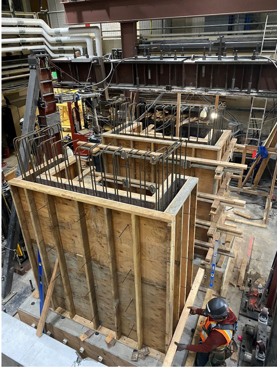
Figure D-12: Phase-II wall formwork
