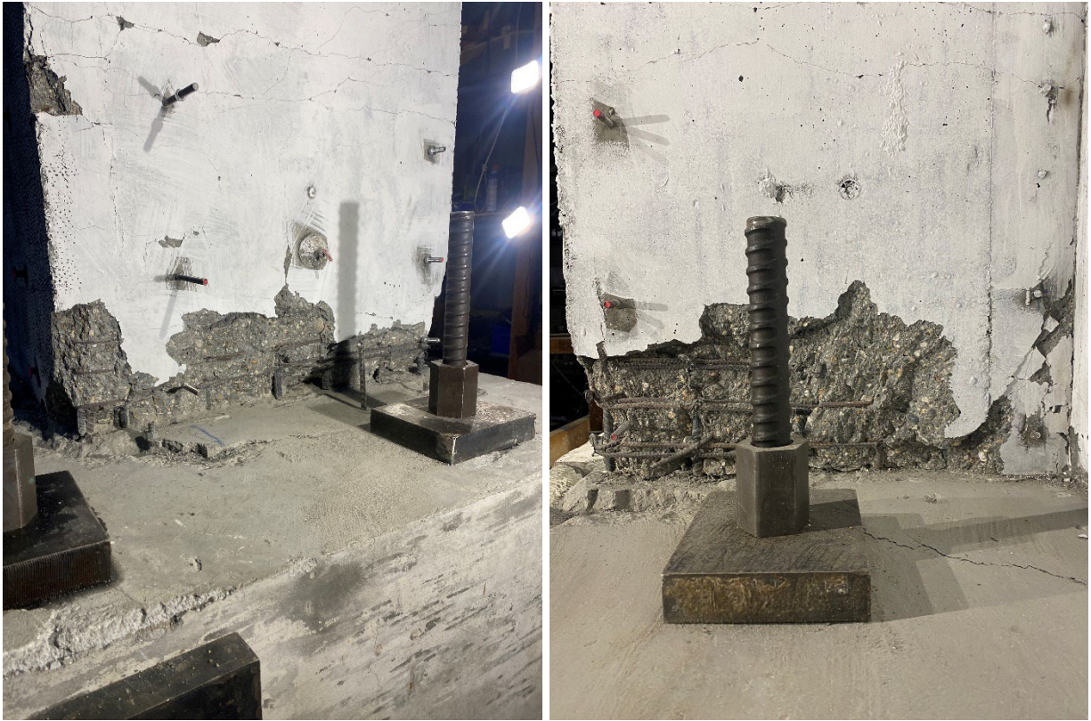
Figure 6-12: East flange outer surface (left) and inner surface (right) after the completion of testing, CW-4
