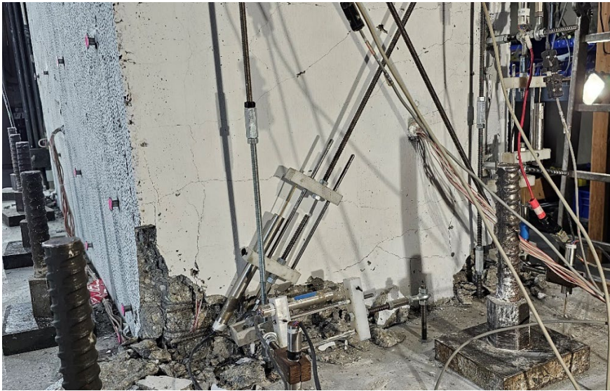
Figure 5-6: East flange after inelastic ramp-down cycles of WLP, CW-2
