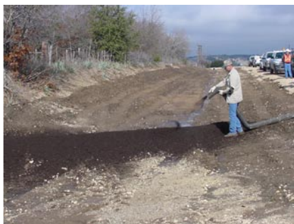
Compost Filter Berm Installation
