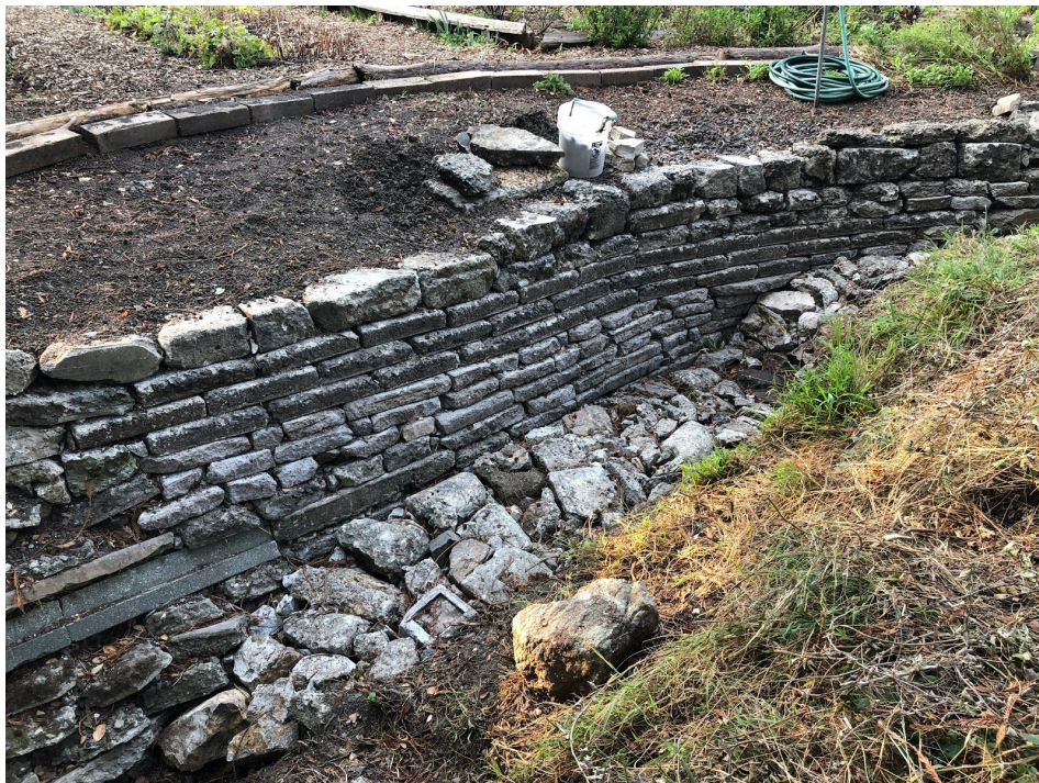
Figure 3: Concrete reinforcement of a portion of the creek.
