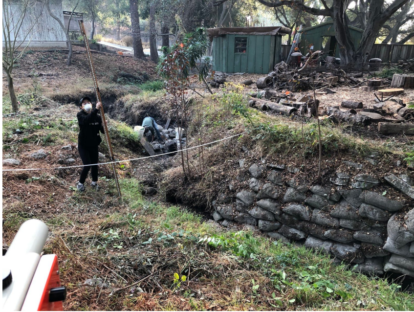
Figure 4: Sac-crete reinforcement of the creek near the recreation area
