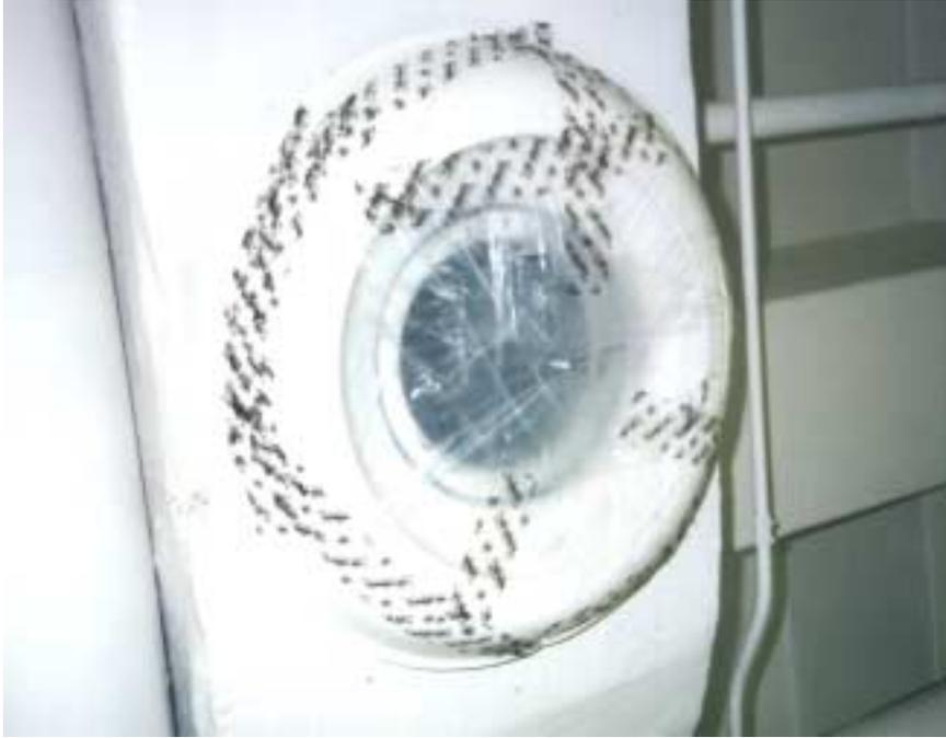
**Figure 3. Sealed diffuser in Building LS-2**
