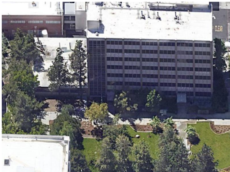
Figure 2.3. JPL 183 Building (source image: Google Maps)
