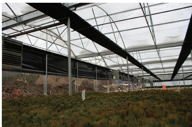
Figure 6.4. A double-layer, polyethylene, gutter-connected greenhouse designed to grow tree seedlings in California. Note the roll-up walls and the black-cloth system for dormancy induction using a shortened photoperiod, with lights to extend the photoperiod.
