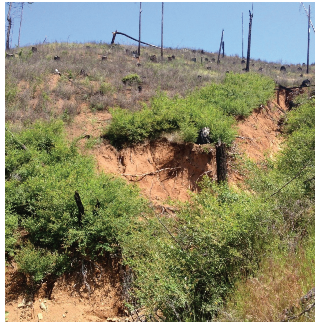
Figure 12.3. Unsprayed vegetative strip on the edge of an eroded feature.
