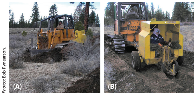
Figure 9.11. A V-blade attached to the front of a crawler tractor (A) scalps away grass and brush, making a level surface of moist mineral soil in preparation for planting 2-0 bare-root ponderosa pine seedlings with the planting machine attached behind the crawler tractor (B).
