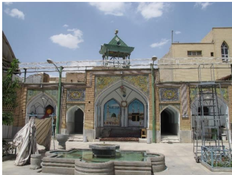
Figure 3-9. The courtyard of the Madraseh-ye Seyyid al-Iraqayn, front showing the northern eyvan and the two side entrances to the courtyard. The metal scaffolding structure running
