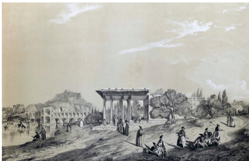
Figure 3-2. A view of the Aynehkhaneh Talar in foreground and the Khawju Bridge in the background, Eugene Flandin, 1840. Source: NY Public Library
