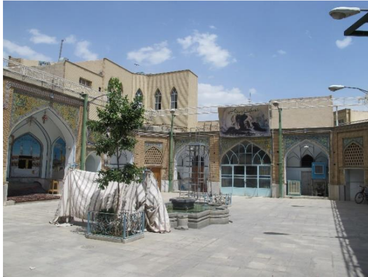
Figure 3-10. The western façade of the courtyard. Photo: Samira Fathi
