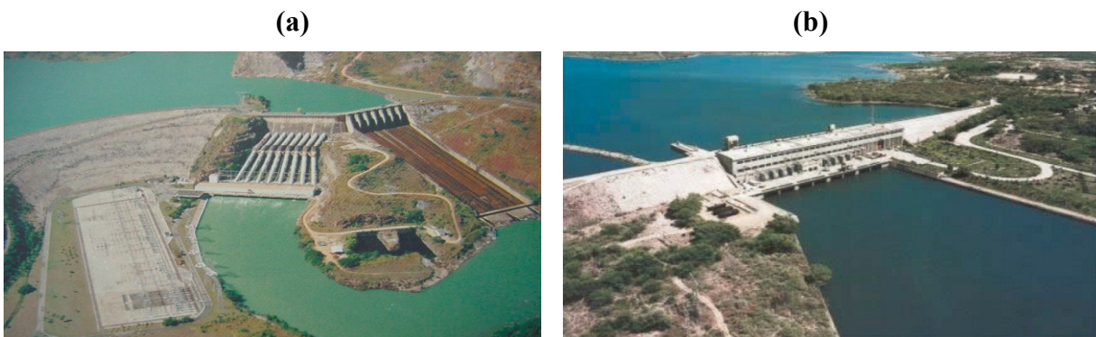
Figure 5-11. General views of (a) Furnas Hydroelectric Dam located on the Rio Grande in Minas Gerais, Brazil [191] and (b) Moxoto Hydroelectric Plant [192].
