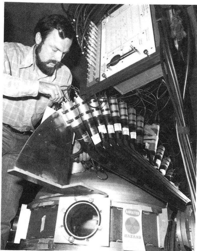
Fig. 5. Hans Gutbrod with the 15 counter tag array and scattering chamber.
