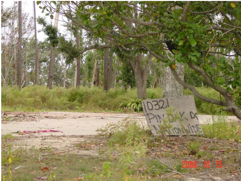
Plate 2 Empty Slab with sign
