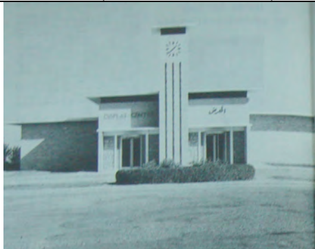
Figure 13. The new Display Center in 1965. (Source: The Kuwaiti )
