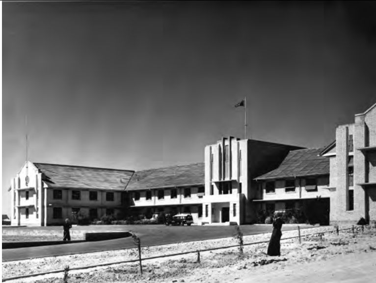
Figure 17. KOC Main Office building. (Source: BP Archive)
