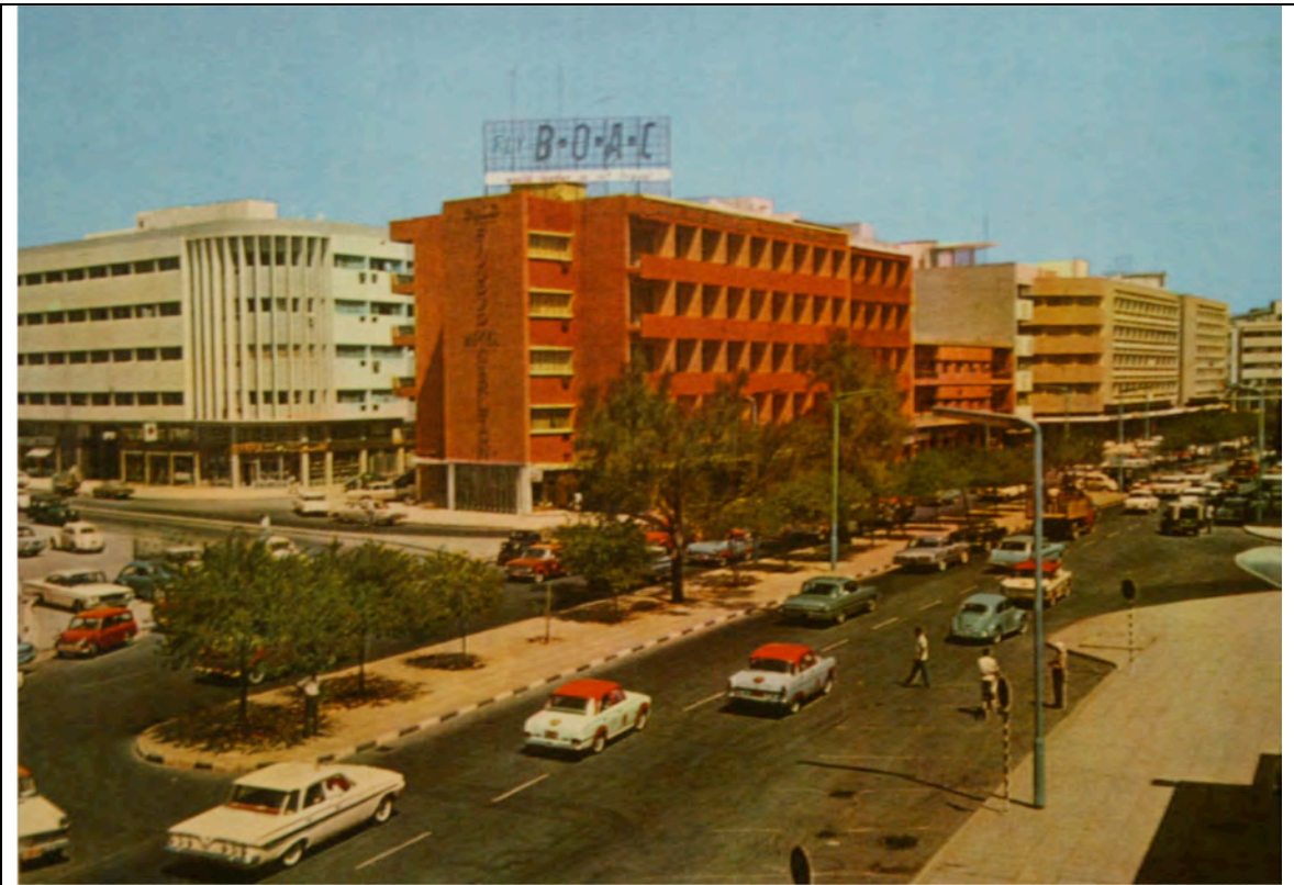
Figure 5. The Carlton Hotel, Kuwait, early 1960s. (Source: Rais)
