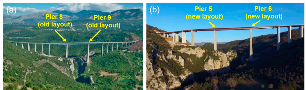
Figure 2. Comparison between: (a) the old (pre-2014) layout and (b) the new (post-2016) layout of the Viadotto Italia (modified from Wikipedia.org, Attribution-ShareAlike 4.0 International, CC BY-SA 4.0 license; https://creativecommons.org/licenses/by-sa/4.0/deed.en , accessed on 26 July 2022).
