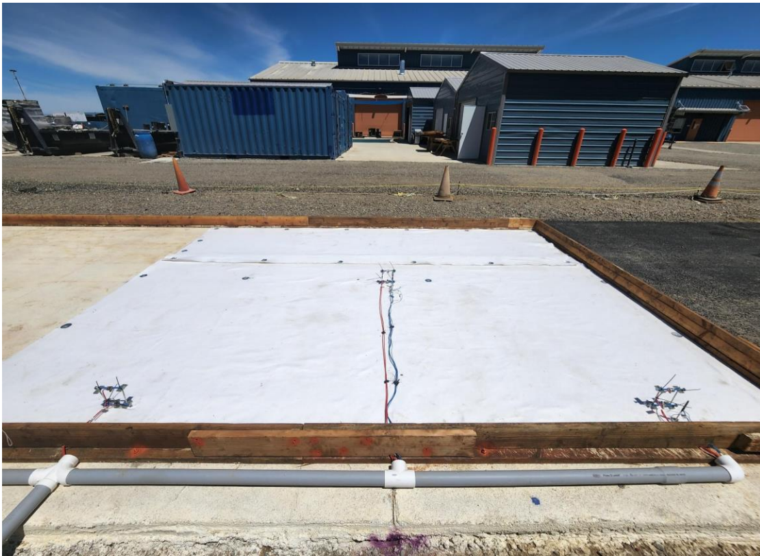
Figure 7-7. Section with geotextile bond breaker, before PLC paving
