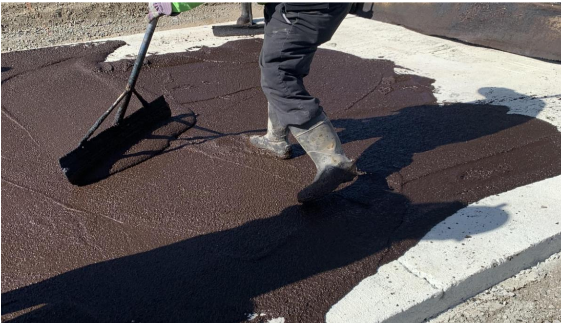
Figure 7-8. Microsurfacing paving
