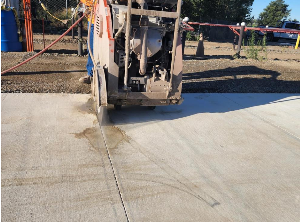
Figure 7-11. Full depth cutting of transverse joints on PLC
