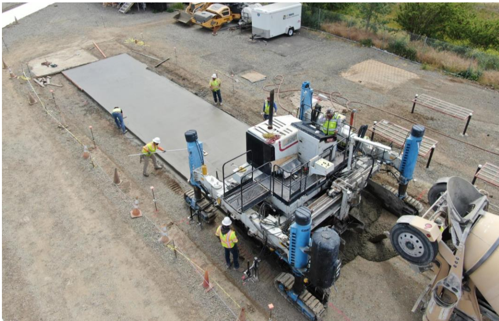
Figure 7-3. LCB construction
