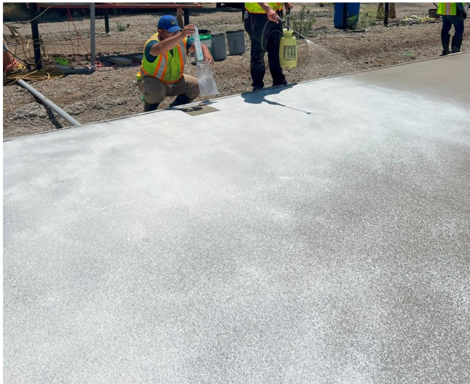
Figure 7-10. Curing compound application on PLC
