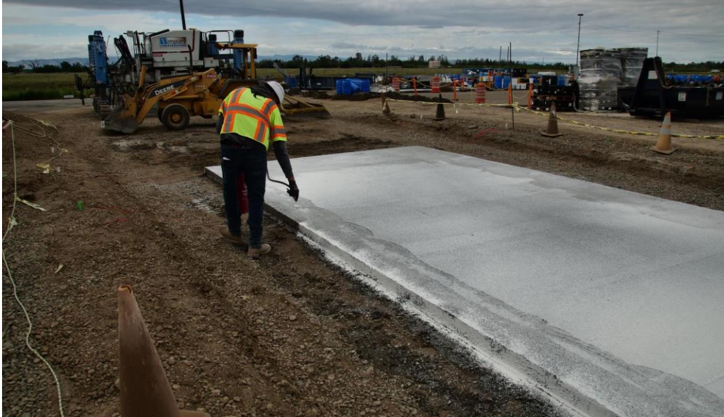
Figure 7-4. Curing compound application on LCB
