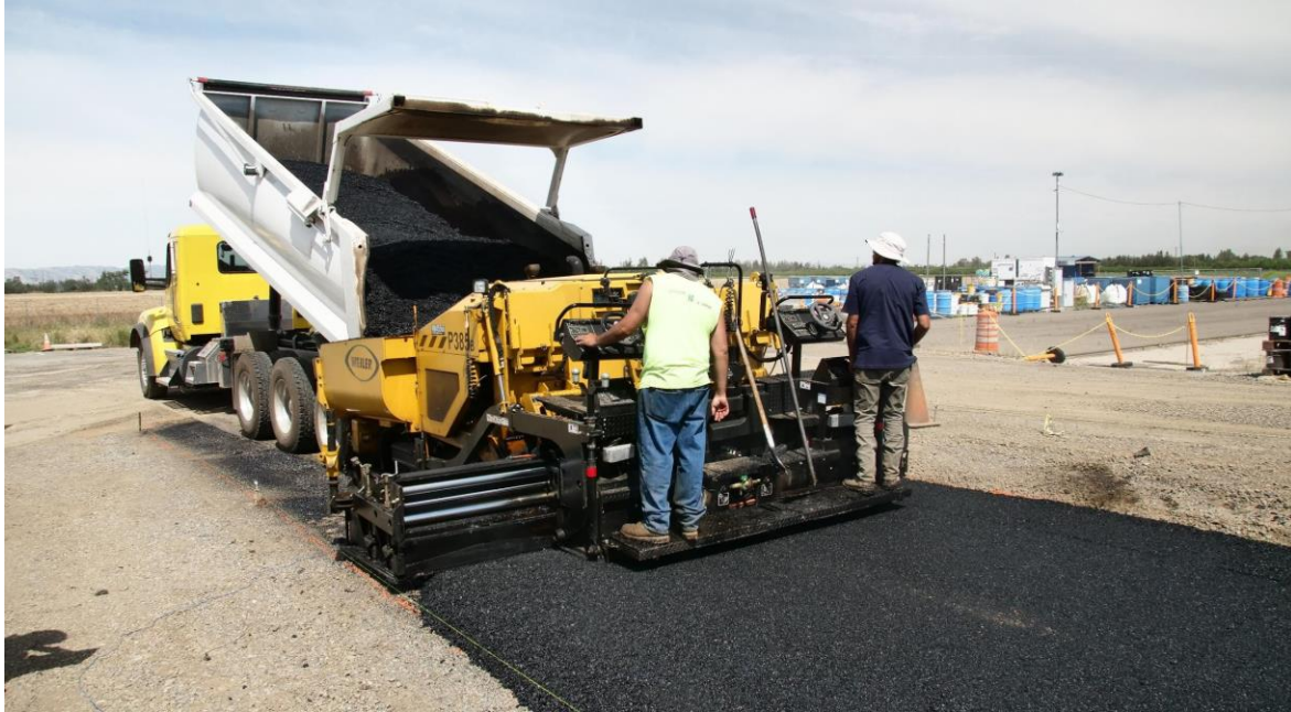
Figure 7-5. RHMA-G paving
