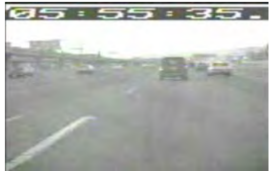
Picture 50: end off ramp split 2
