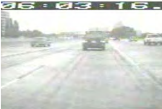
Picture 35: End on ramp junction 3
