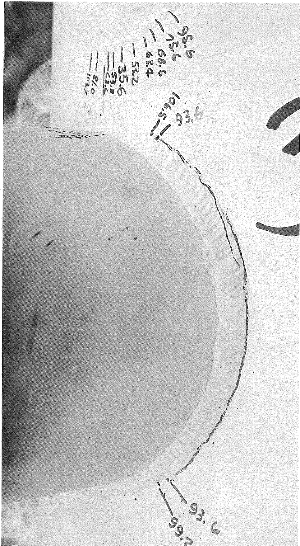
FIG 18 JOINT TYPE I - SPECIMEN No. 3 DETAILED CRACK PROPAGATION IN COLUMN MEMBER WALL
