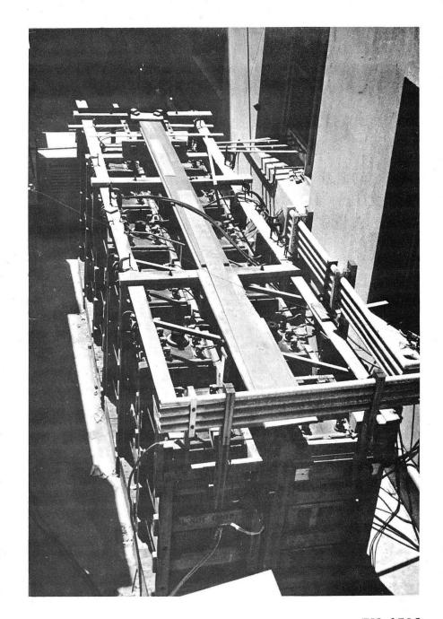
Fig. 20. The 20,000 ampere-hour submarine storage batteries, which energize the A and B magnets.
