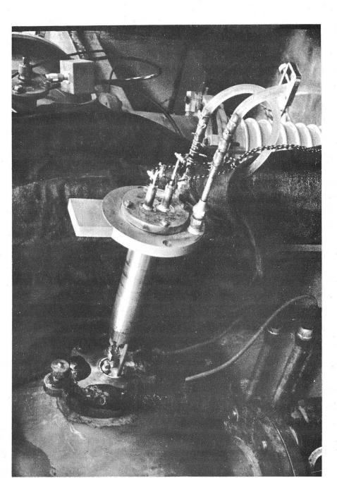
Fig. 23. Placing the electron bombardment oven loader in the apparatus.
