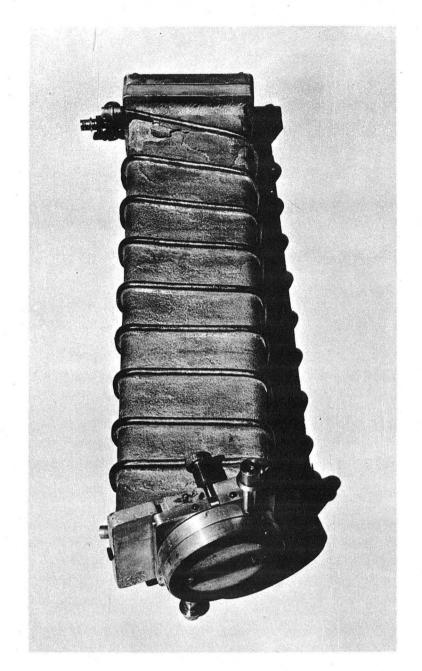
Fig. 22. The bell jar used to bombard gaseous xenon with protons.
