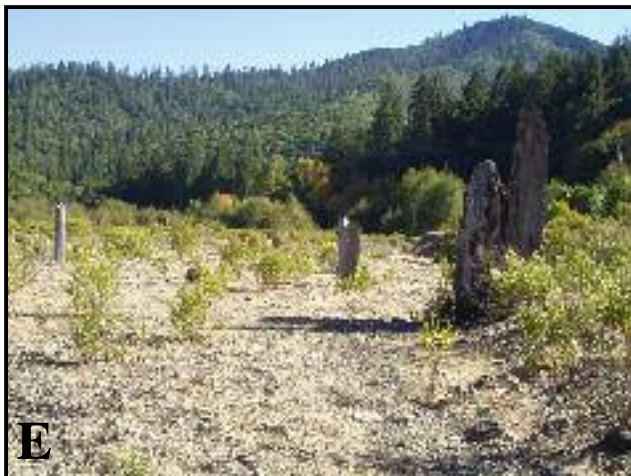
Figure 10: Remnants of Channel Reconstruction Project. A) Abandoned channel B) Suspected remnants of rock and log revetment; C) Suspected remnants of vortex rock weir; D) Active channel looking downstream; E) Vertically placed logs in floodplain that are remnants of debris flow regulation structures.
