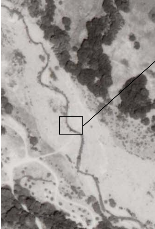
a) Constructed Channel
