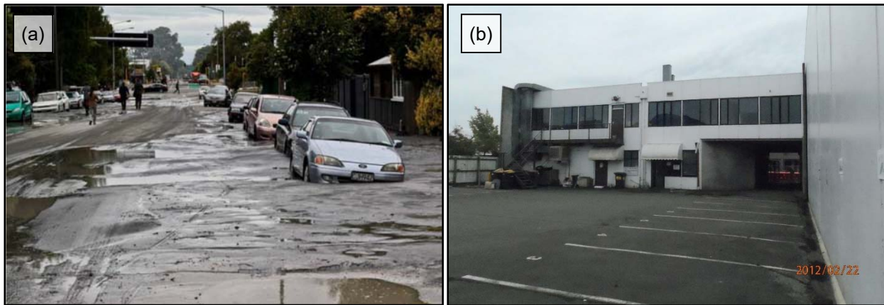
Figure 4.1: (a) Liquefaction Site (from GEER Report No. 27), and (b) No-liquefaction Site (from Mr. Rick Wentz of Wentz-Pacific, Ltd.) in Christchurch.
