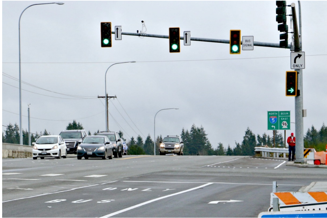
Transit queue jump on 128 th St SW in South Everett. Source: Fesler, 2018
