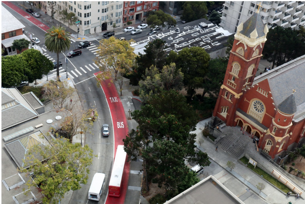
Intersection of O'Farrell and Franklin Street in San Francisco. Source: Wambeke and Wambeke, 2016
