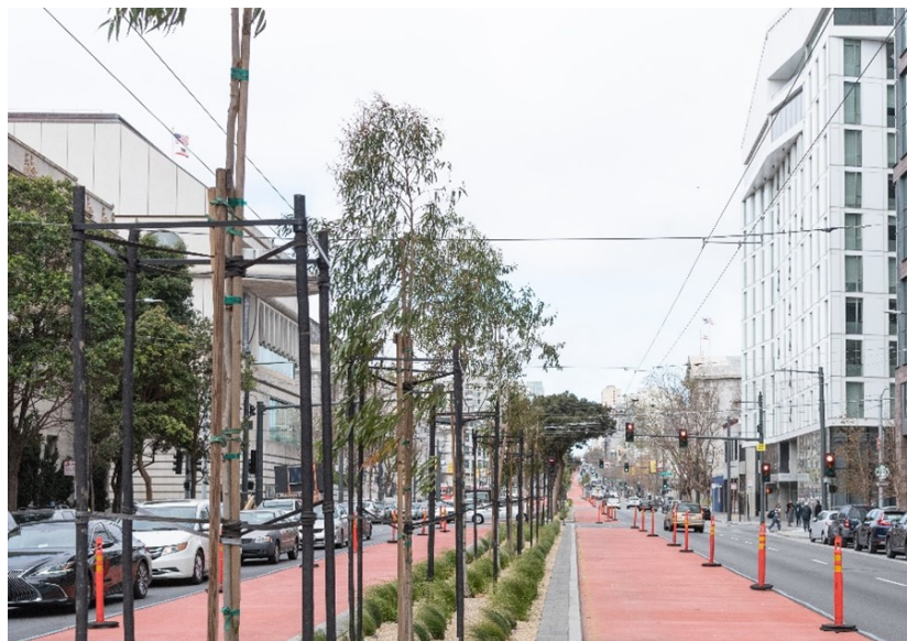
The Van Ness Bus Rapid Transit bus lanes. Source: Gravener, 2022
