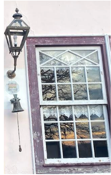
Figure 46. Detail of the windows.
