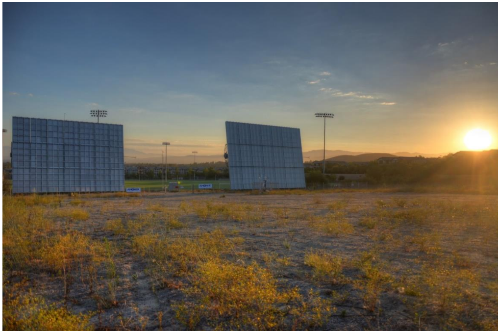
Figure 43. 74 kW concentrated PV systems installed on the UCIMG.
