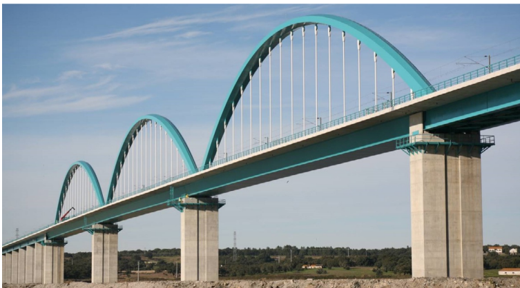
Fig. 18.2 Overview of the bridge over the Sado River.
