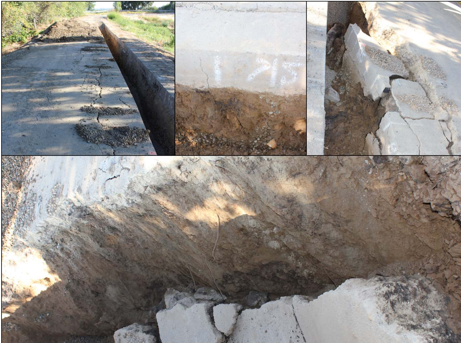
Figure 3-124. Station TT 65 to TT 88 failed under equipment loading during repair. Dark staining appearing to be manganese oxides appear along the failure plane in numerous locations indicating possible pre-existing fracturing within the leve
