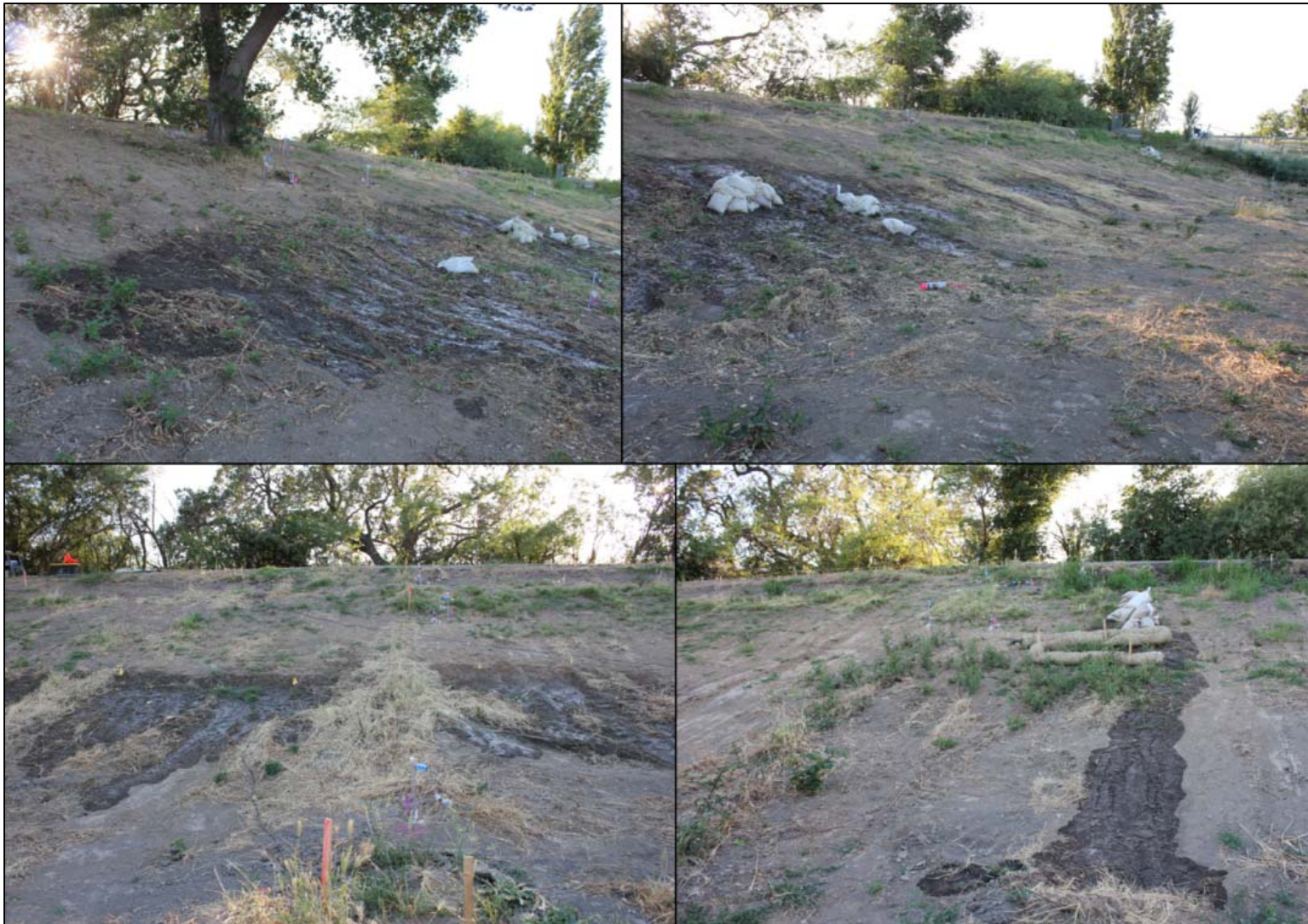
Figure 3-146. Flow on the landside at the end of the dye test (Time = 245.1 hours).
