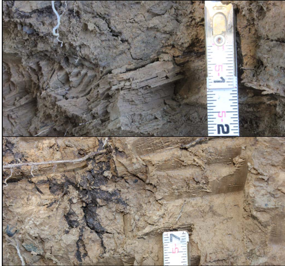
Figure 3-125. Trench wall failure at Stations 65 to 88. Close in view at Station 75 shows fractures focused within weak zones of Material 2, thinly bedded sandy silt (top), and zones stained with manganese oxide, indicating previous fractures (bottom).
