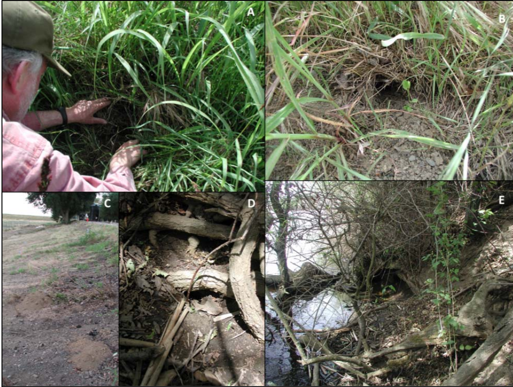
Figure 3-13. Evidence of burrowing animals on the landside consisting of voles (A and B) and gophers (C) and evidence of muskrats found on the waterside (D and E).
