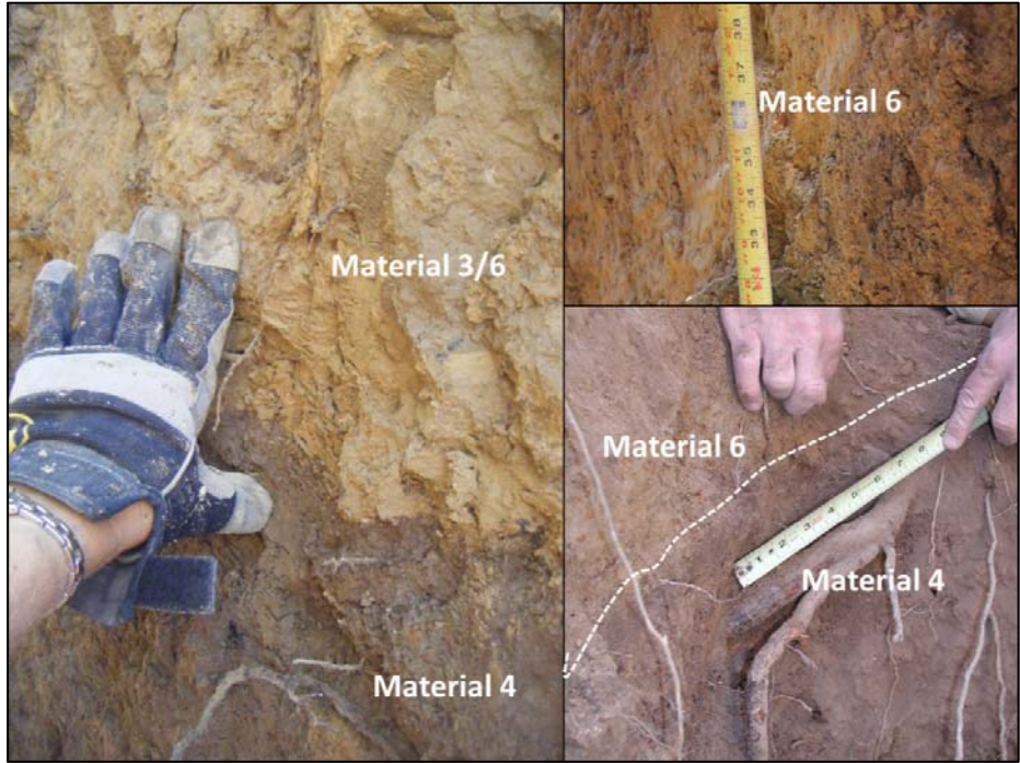
Figure 3-45. Pockets of Materials 3 and 6 (light brown and olive sandy silts, respectively) frequently occur together (left) and underlain by the plastic silt layer, Material 4.
