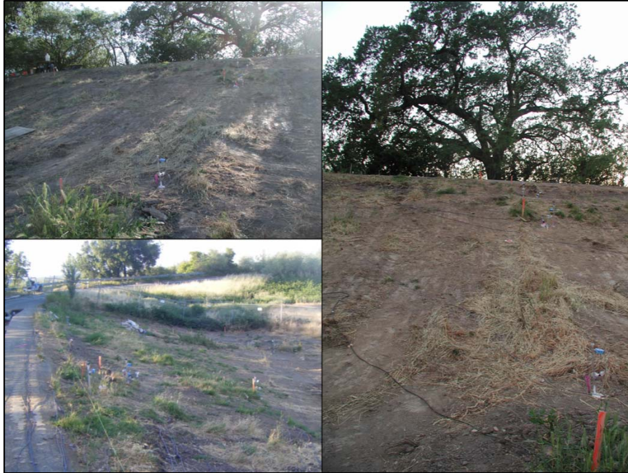
Figure 3-93. Instrument Line B at waterside oak tree looking west (upper left, right) and north (lower left).
