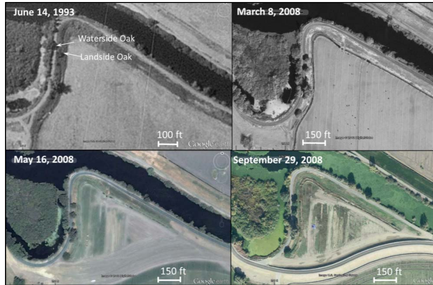
Figure 3-18. Image of the study site in 1993 showing a small, but present, landside oak. Images between March and September of 2008 show the construction of the levee bypass.
