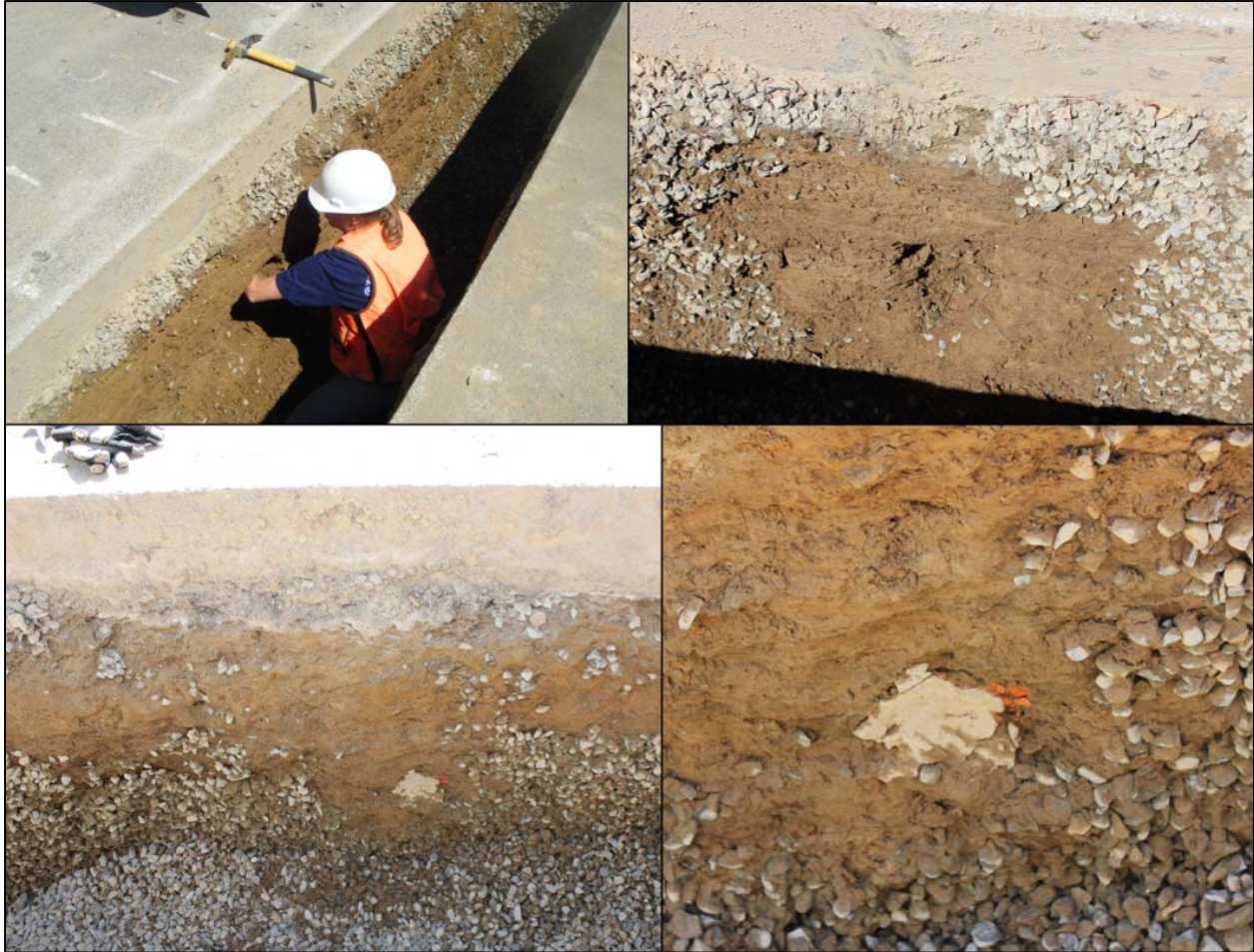
Figure 3-181. Open burrow at waterside Station CT 11 (top images) and intact patch on burrow at landside Station CT 12 (bottom images).
