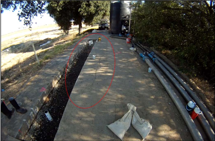
Figure 3-122. Crack at Stations TT 70 to 95 seen through wide angle lens on 5/31/12 facing south. Cracking observed during original excavation but grew slightly (<math><1/8''</math>) during flow testing.
