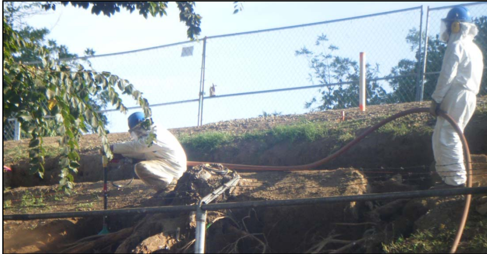
Figure 2-80. View of air knife operation during post-flow test site characterization effort.
