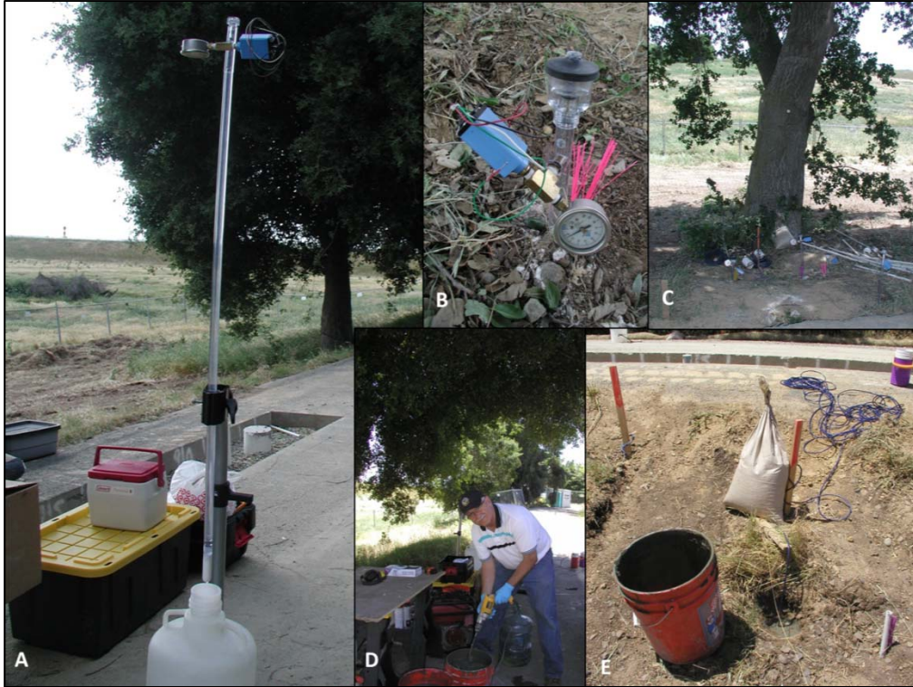
Figure 3-90. Tensiometer is leak-checked, saturated (A) and sealed into the ground (B and C). Grout is mixed (D) and piezometers are grouted into the ground (E).
