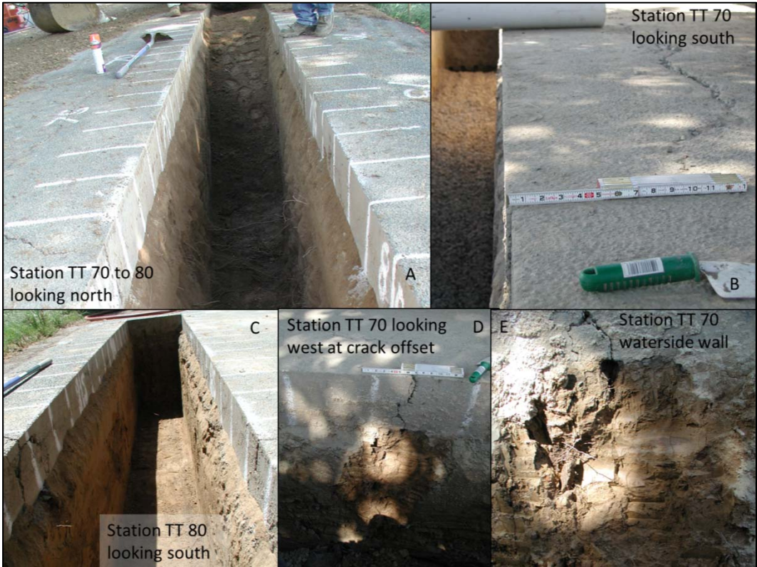
Figure 3-122. Crack at Stations TT 70 to 95 seen through wide angle lens on 5/31/12 facing south. Cracking observed during original excavation but grew slightly (<math><1/8''</math>) during flow testing.
