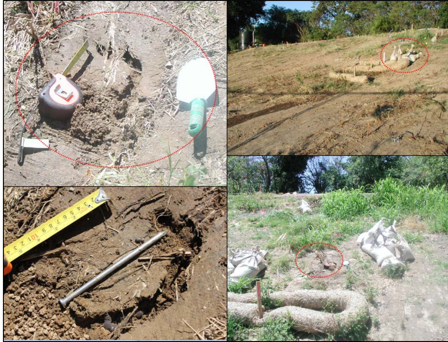
Figure 3-171. The gravel bags were parted (lower right) and a single burrow was revealed at Station CT 7. The burrow was about 1 ½ inch in diameter and the top of the burrow extended into the slope.
