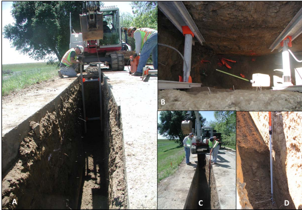
Figure 3-34. A) The control trench is shored for logging; B) Station 26 to 31.5 is shored for manual excavation and logging of first large roots; C) and D) Smaller roots are logged and trimmed from above prior to proceeding with excavation.
