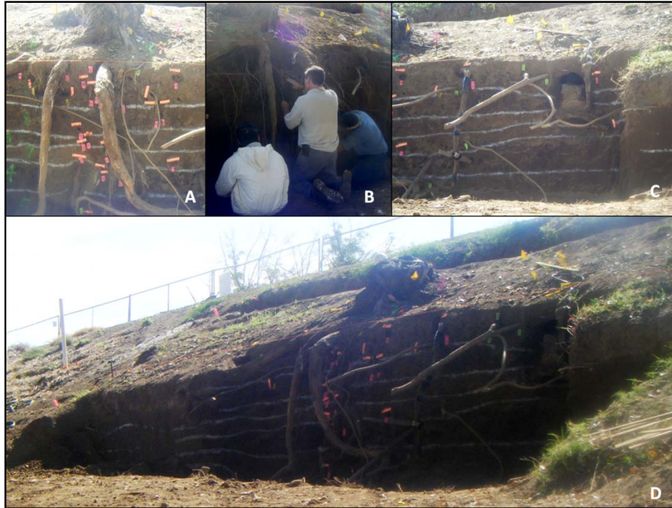
Figure 2-85. Slice 1 wall surface
