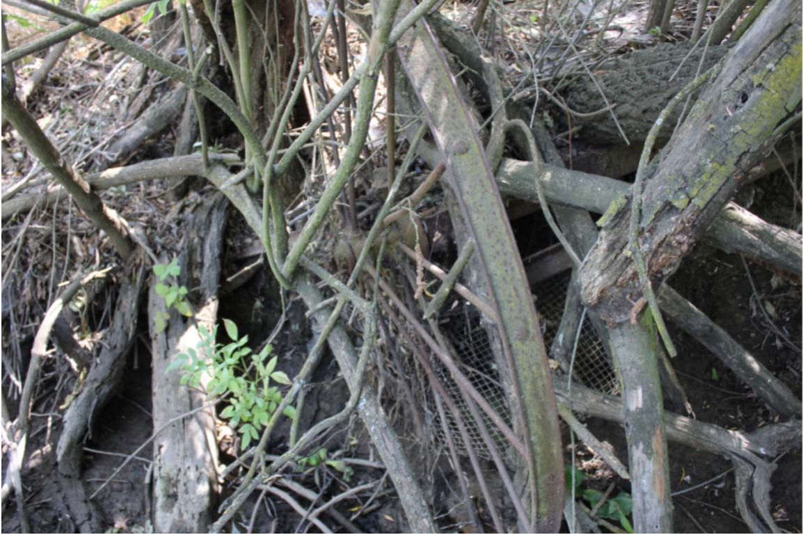
Figure 3-28. The wheel of what appears to be horse-drawn farming equipment protruding from the waterside of the levee (Sta TT 70). The axle and possibly the other wheel extend into the levee slope.
