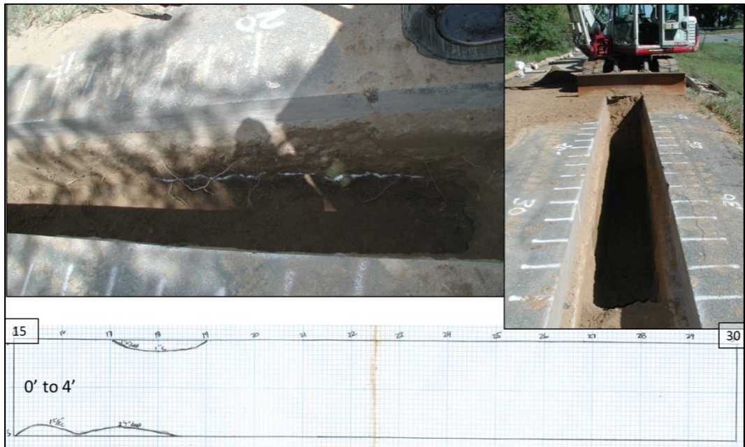
Figure 3-56. Root log at 0 to 4 foot depth Station TT 15 to 30.
