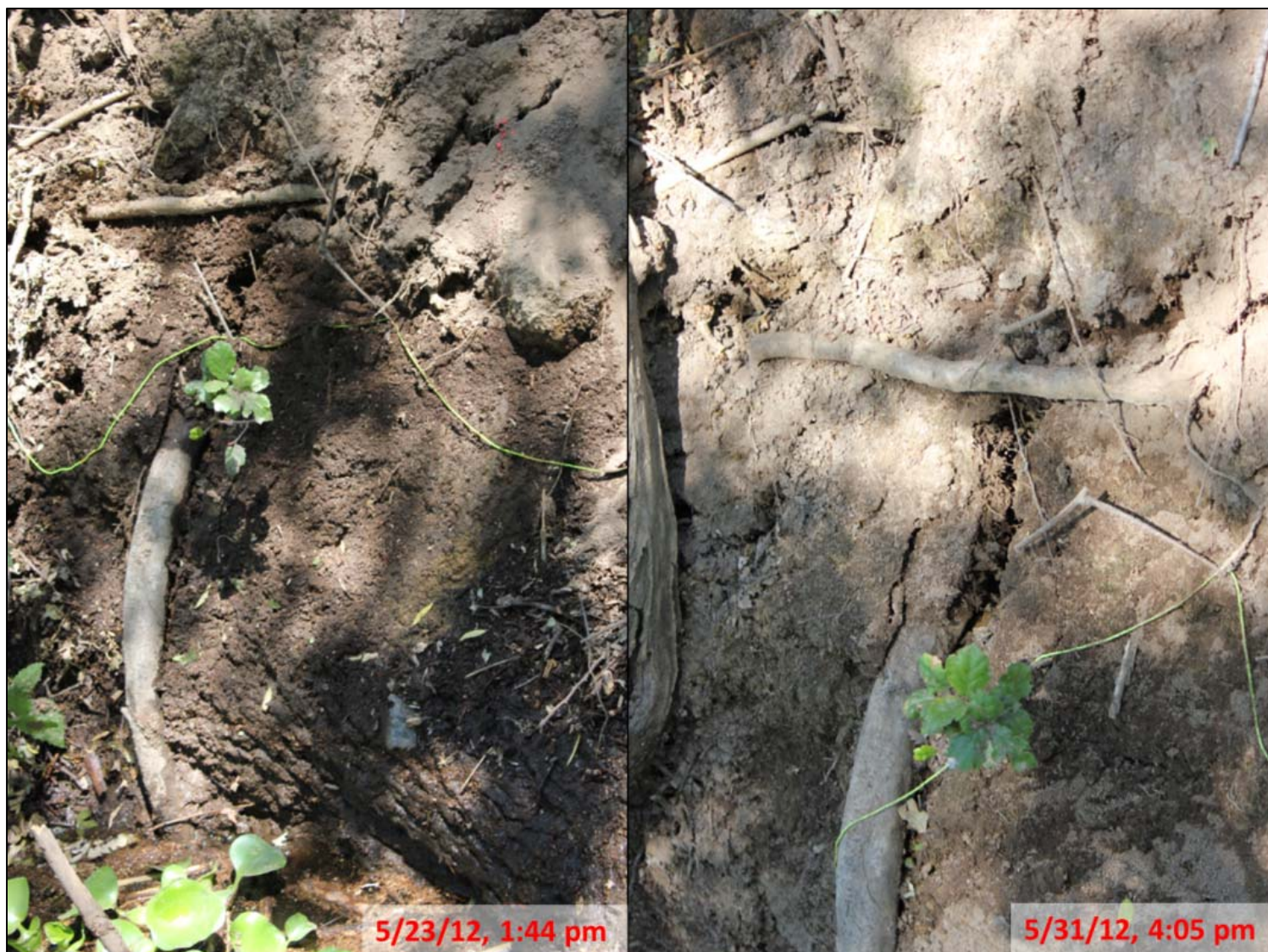
Figure 3-147. Several hours into the dye test, early seep discovered at waterside oak ceased flowing once the tree fell (left) and did not begin flowing again during the dye test on 5/31 (right).
