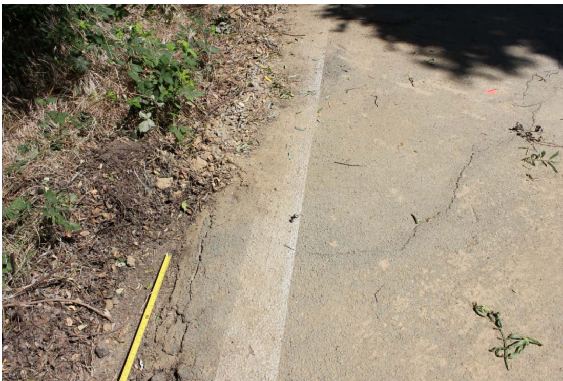
Figure 3-120. Cracking was observed in the pavements at approximate Stations TT 70 to 95 at 6 pm on the second day of the flow test (Time = 28.3 hours).
