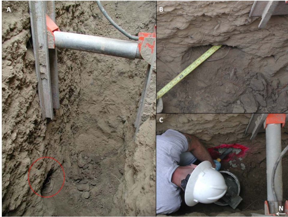
Figure 3-74. Burrow on landside of Station TT 57 at 7 foot depth. Vegetative debris and live root growth found inside 2 ½ diameter hole (left, top right). A plug of grout is placed (bottom right).
