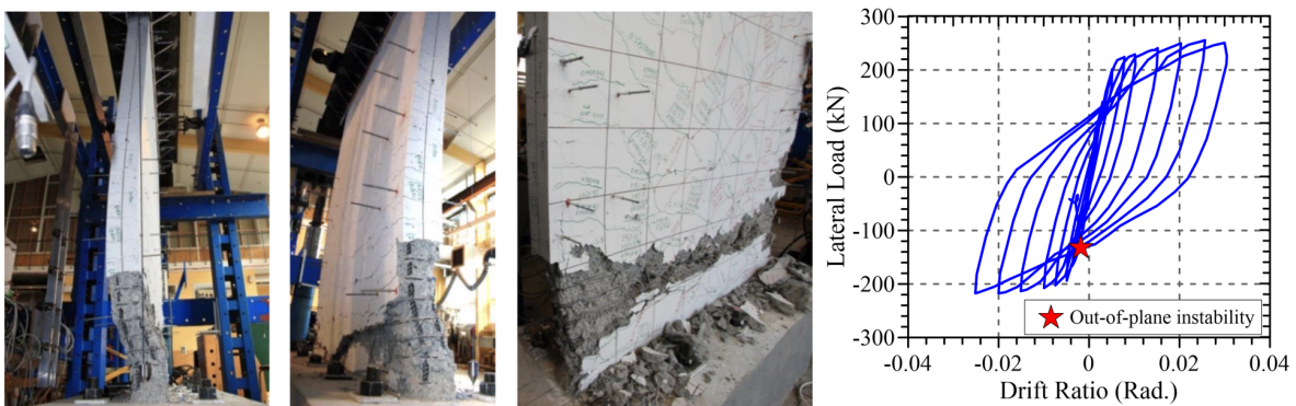
(a) Damage at the end of testing
