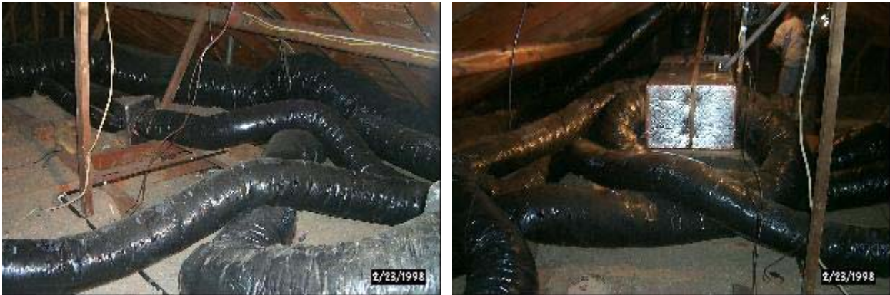
Figure 13. Second and final installed retrofit of ductwork after being moved to attic floor and before adding insulation.
