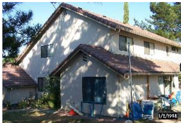
Figure 2(b). Exterior side view of Concord test residence showing gable attic vents and existing outside AC condenser unit placement [lower left].
