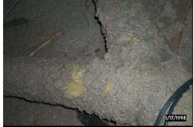
Figure 5(b). Existing insulated metal duct splitter and insulation coverage.
