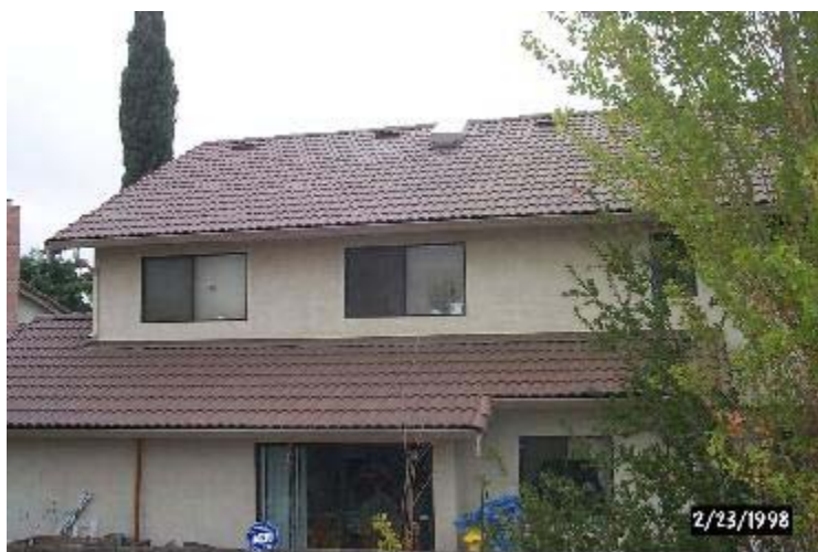
Figure 2(c). Exterior rear view of Concord test residence.
