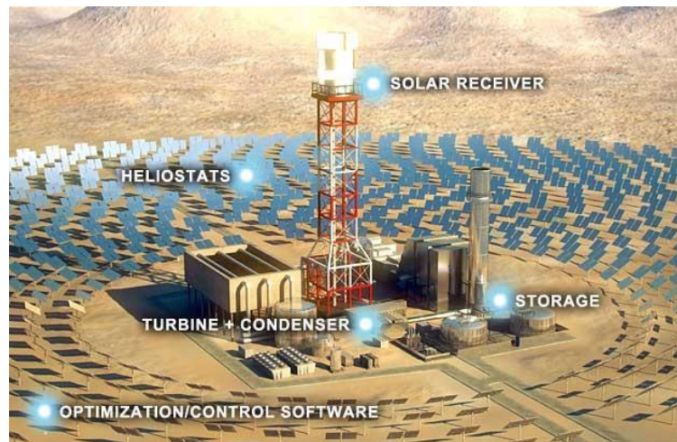
Figure 1.11 Schematic diagram and picture of the power tower system. (Image sources : http://www.brightsourceenergy.com/ )
