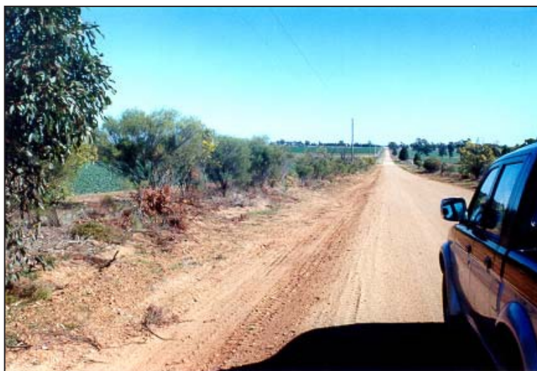
Figure 3. A typical narrow 20.12 m (1 chain) road reserve in southern NSW where a gravel road and adjacent table drains have been recently graded as part of a regular maintenance program. In the process, all previous vegetation (approx 2 m x 1.7 km) has been removed, apart from a narrow strip of native vegetation (mostly Acacia and Senna species) along the fenceline.
