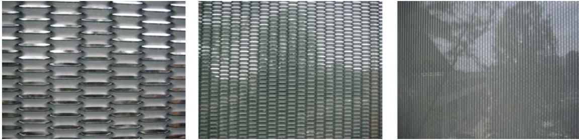
Figure 11.11 Revitalisierung Haupthaus KfW, Frankfurt (Architekten Theiss and ip5 ingenieurpartnerschaft, 2003 - 2007). Images taken looking through a moveable exterior metal panel at varying distances (0.2, 1, 3 meters). The panel consists of glass, expanded metal, and a PVB interlayer.
