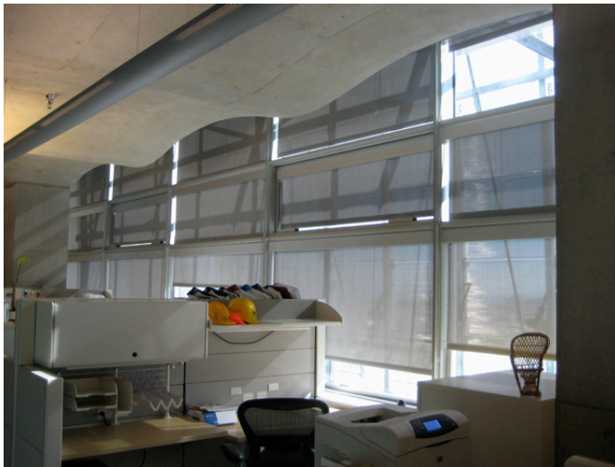
Figure 5.14 Example perimeter workstation adjacent to the SE facade showing location of interior roller shades. Image taken on November 1st at 10:20 AM PST.
