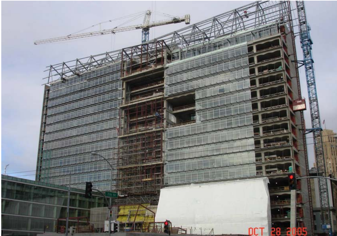
Figure 3.8 Floor to ceiling high glazing with high visible light transmittance on SE facade photographed prior to installation of exterior perforated steel scrim. From McConahey (2005).
