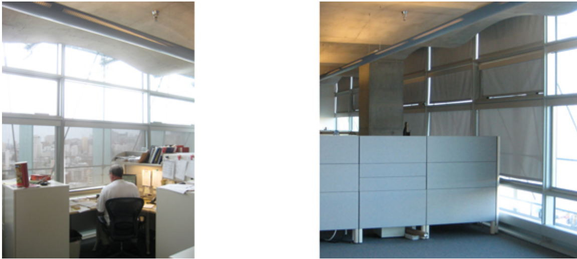
Figure 5.2 Overview of NW facade workstations where interior roller shades were added to the row of vision windows only (left) and to the upper two rows of windows in addition to the vision windows (right). The openness factor for shades in both images is the same (5%). The difference in perceived transparency is the result of different camera exposure settings.
