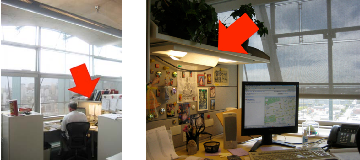
Figure 10.9 Location of task lighting installed in workspace partitions on NW (left) and SE (right) perimeter zones. Note occupant intervention for glare control in righthand image.
