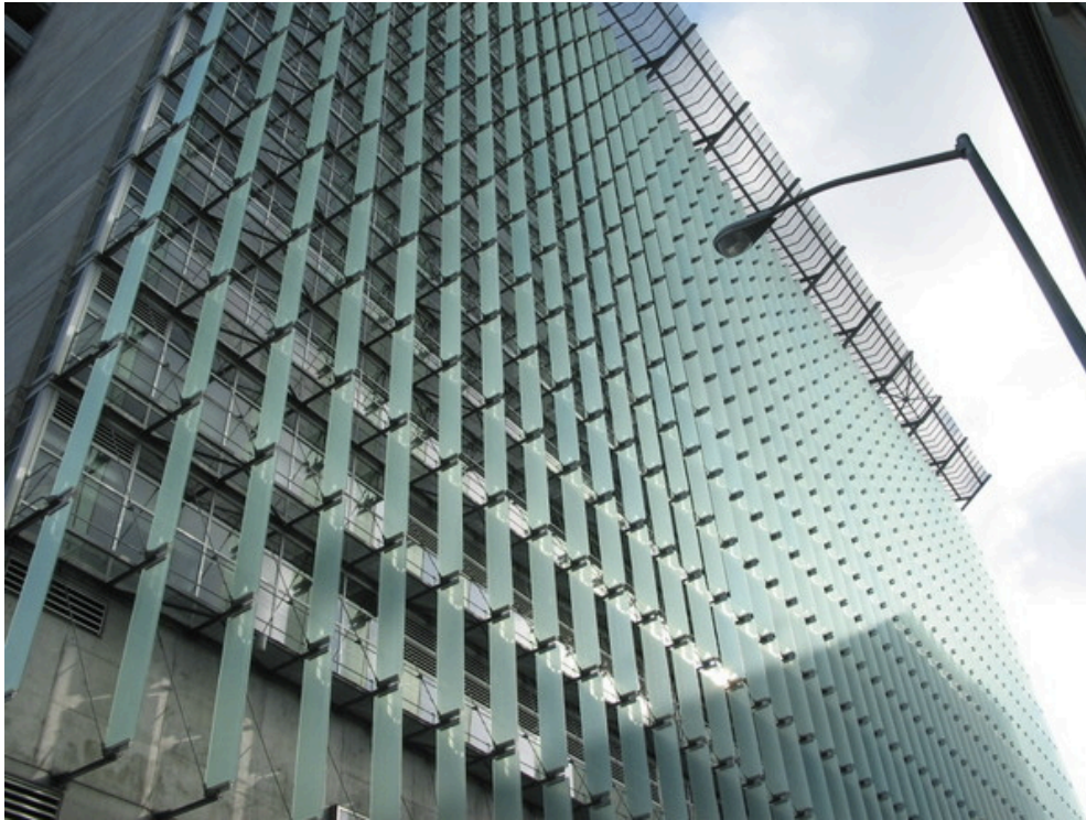
Figure 3.12 Exterior view of the NW facade exterior solar shading devices. 14
