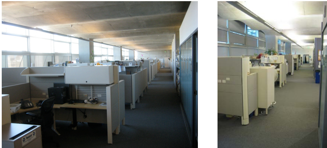
Figure 10.3 Typical perimeter lighting zone on the NW (left) and SE (right) sides of the SFFB. NW perimeter lighting zones include two rows of workspaces parallel to the facade.
