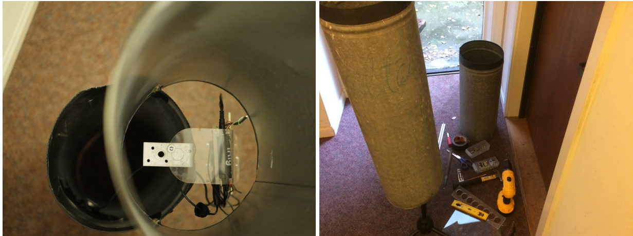
Figure 44. Left: mounting L-bracket for stand and acrylic plate. Right: measuring, bolting, and cutting the air ducts.
