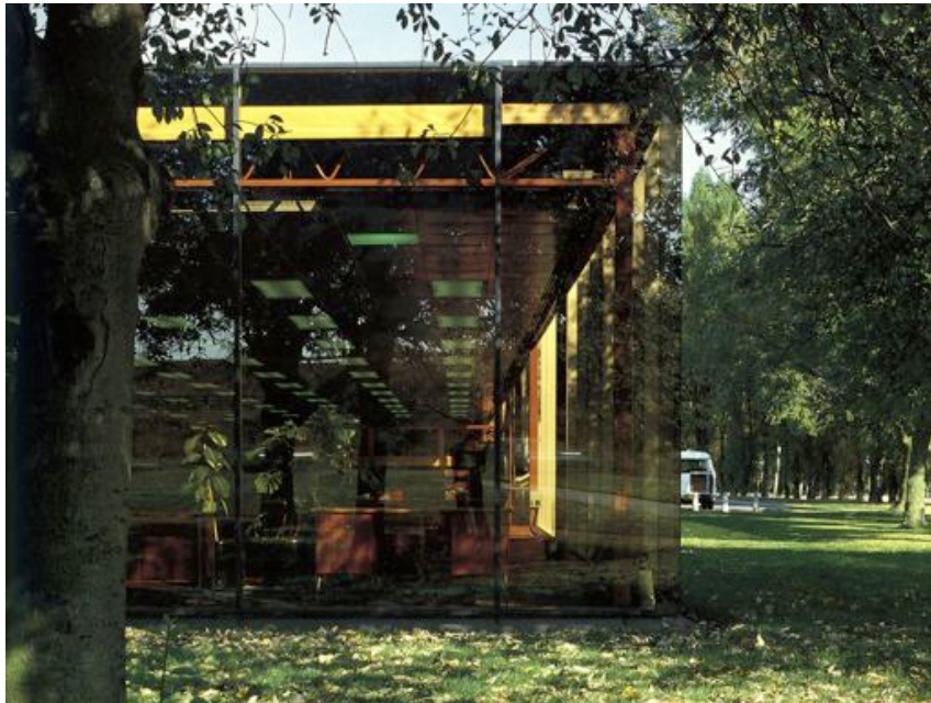
Fig. 3.21: Norman Foster, IBM Pilot Head Office, Cosham (1970)
