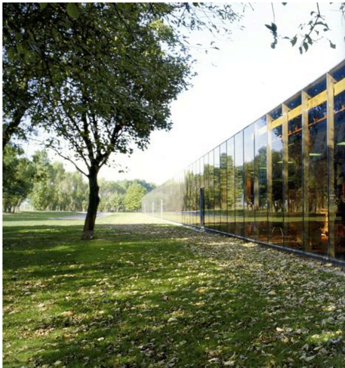
Fig. 3.12: Norman Foster, IBM Pilot Head Office, Cosham (1970)
