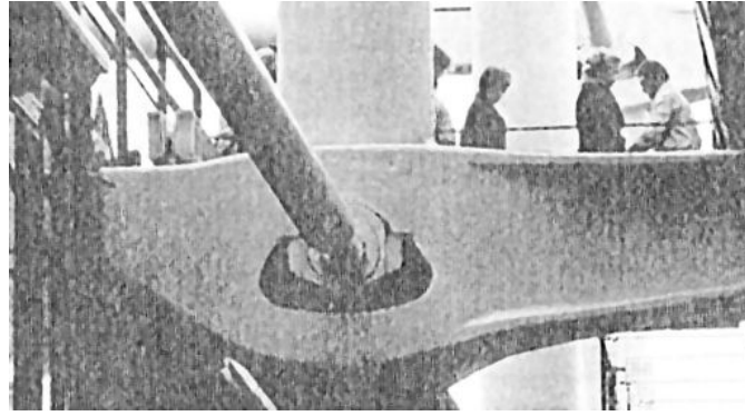
Fig. 3.20: Peter Rice, gerberette detail. From Peter Rice, An Engineer Imagines (London: Artemis, 1994).
