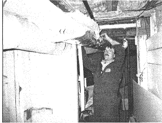
Installing Duct Wrap
