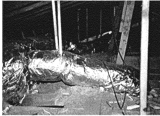
After adding duct insulation
