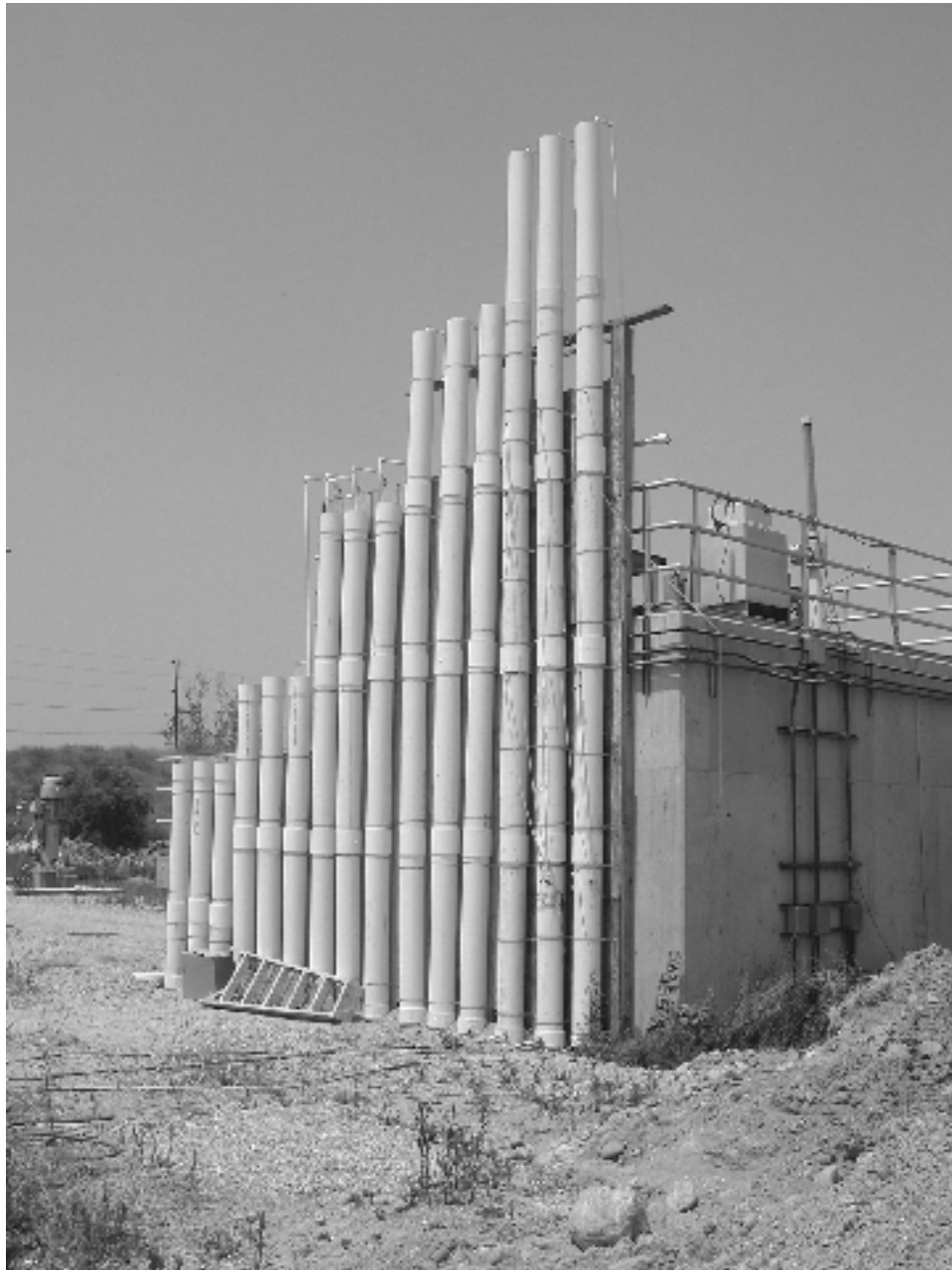
Figure 6. MODIFICATION 2 COLUMNS IN PLACE AT RIX
