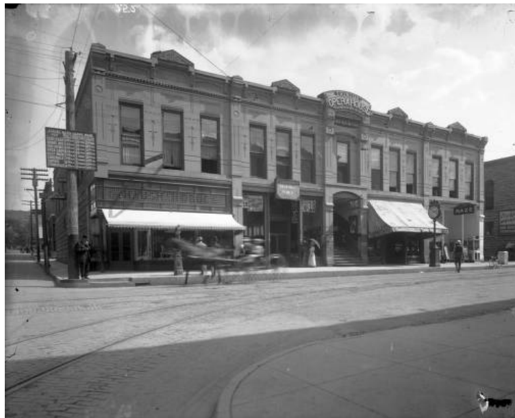
Figure 17. Trinidad Opera House (1905-1915), Denver Public Library Digital Collections, https://digital.denverlibrary.org/digital/collection/p15330coll21/id/11366/rec/5 .
