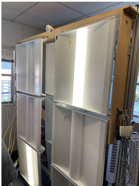
Figure 4. Picture from the PoE lighting rack test setup in LBNL's FLEXLAB.
