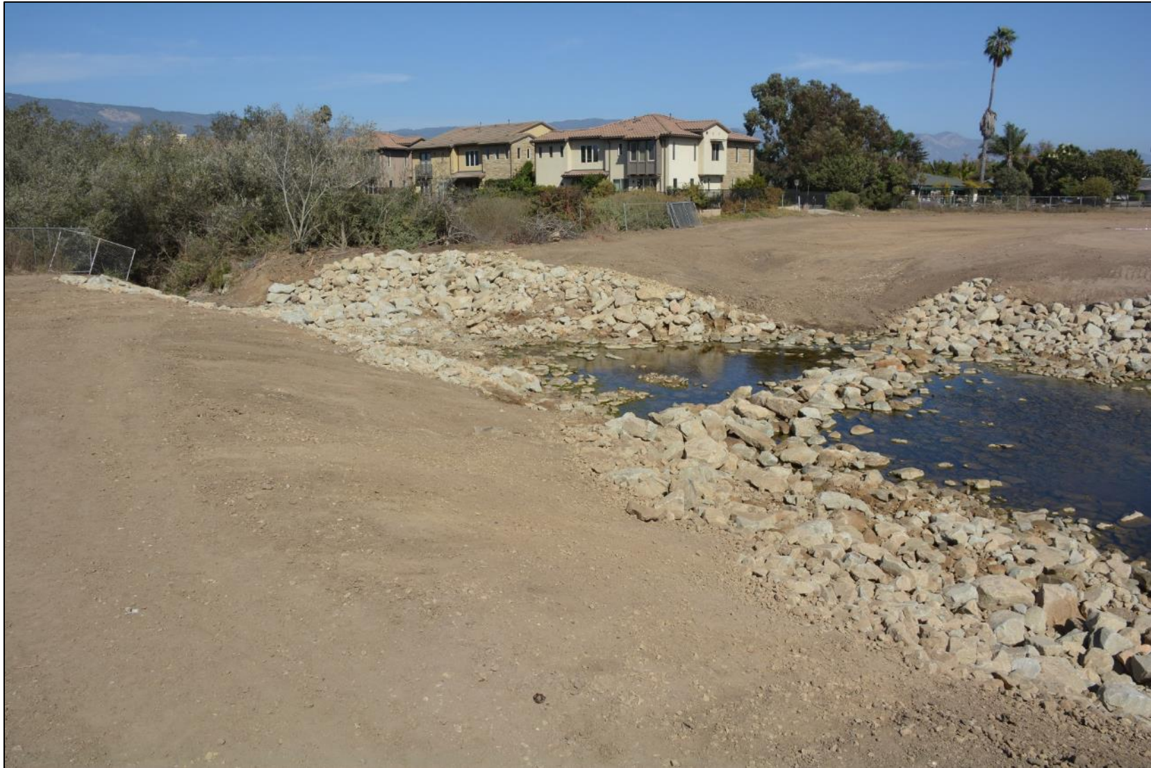
Baseline photo – post-grading, October 10, 2017.
