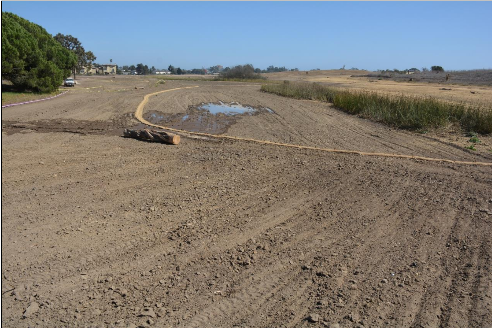
Baseline photo – post-grading, October 10, 2017.
