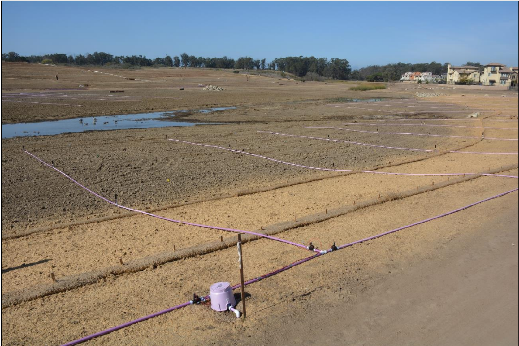
Baseline photo – post-grading, October 10, 2017.
