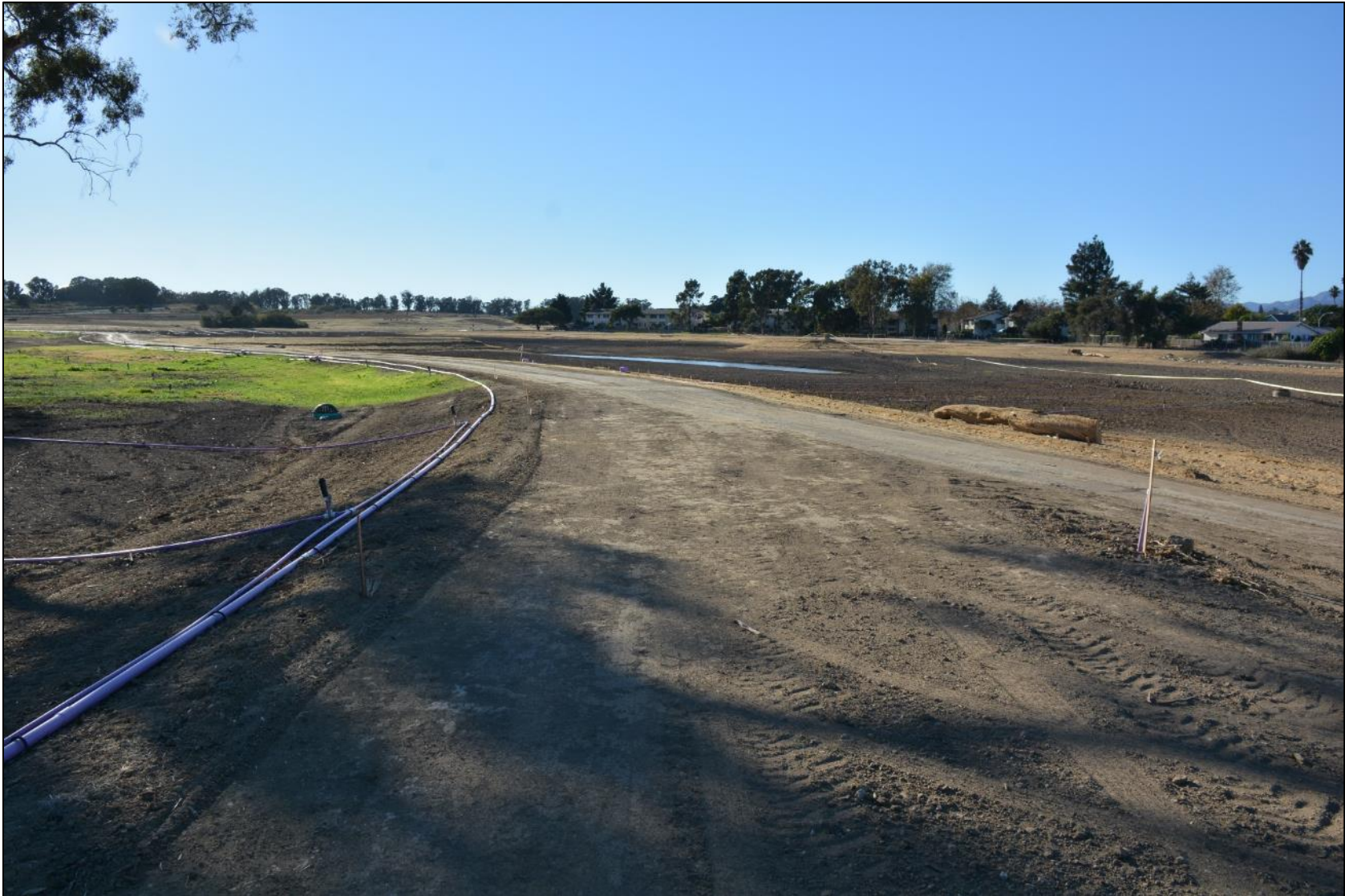
Baseline photo – post-grading, October 24, 2017.
