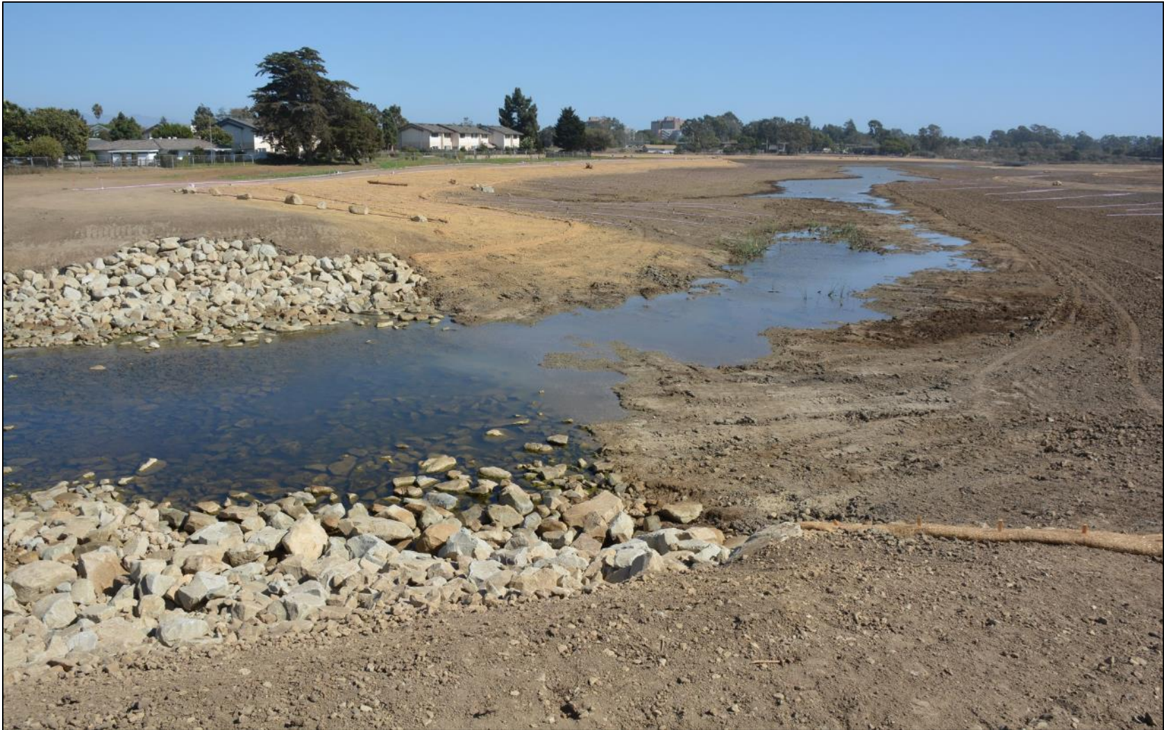
Baseline photo – post-grading, October 10, 2017.
