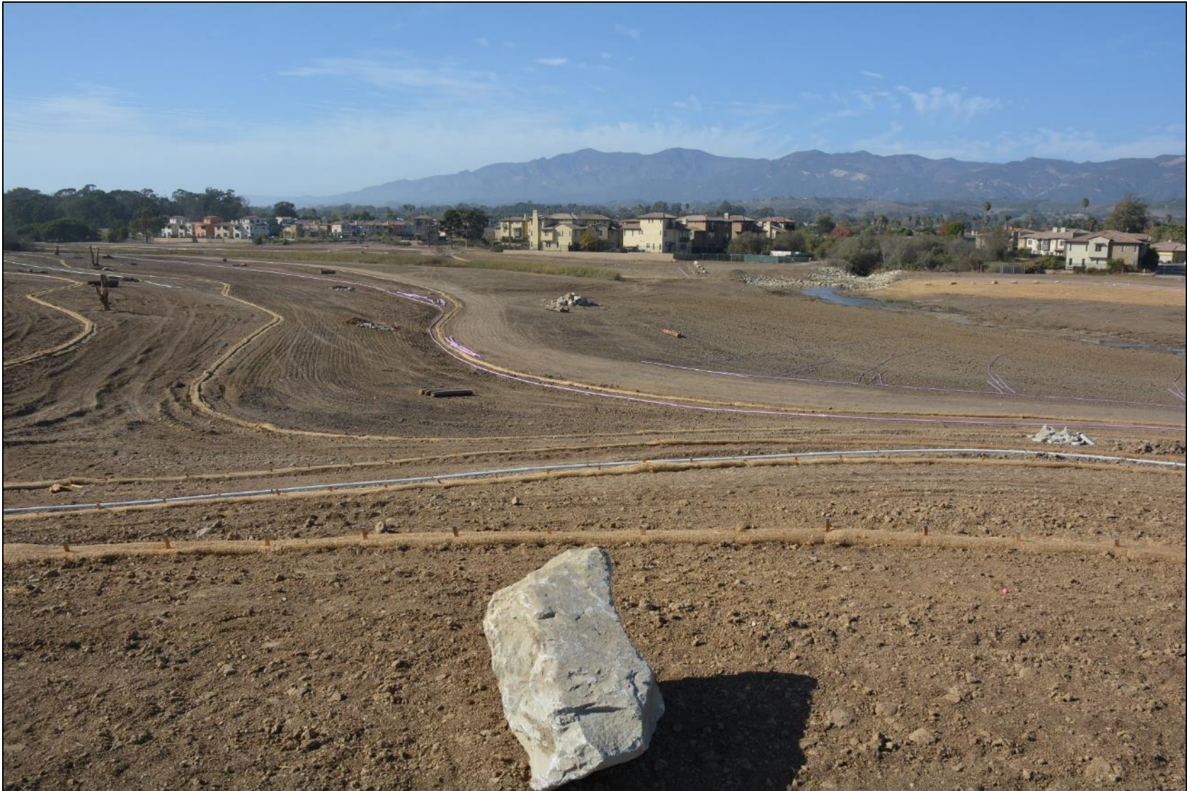
Baseline photo – post-grading, October 10, 2017.
