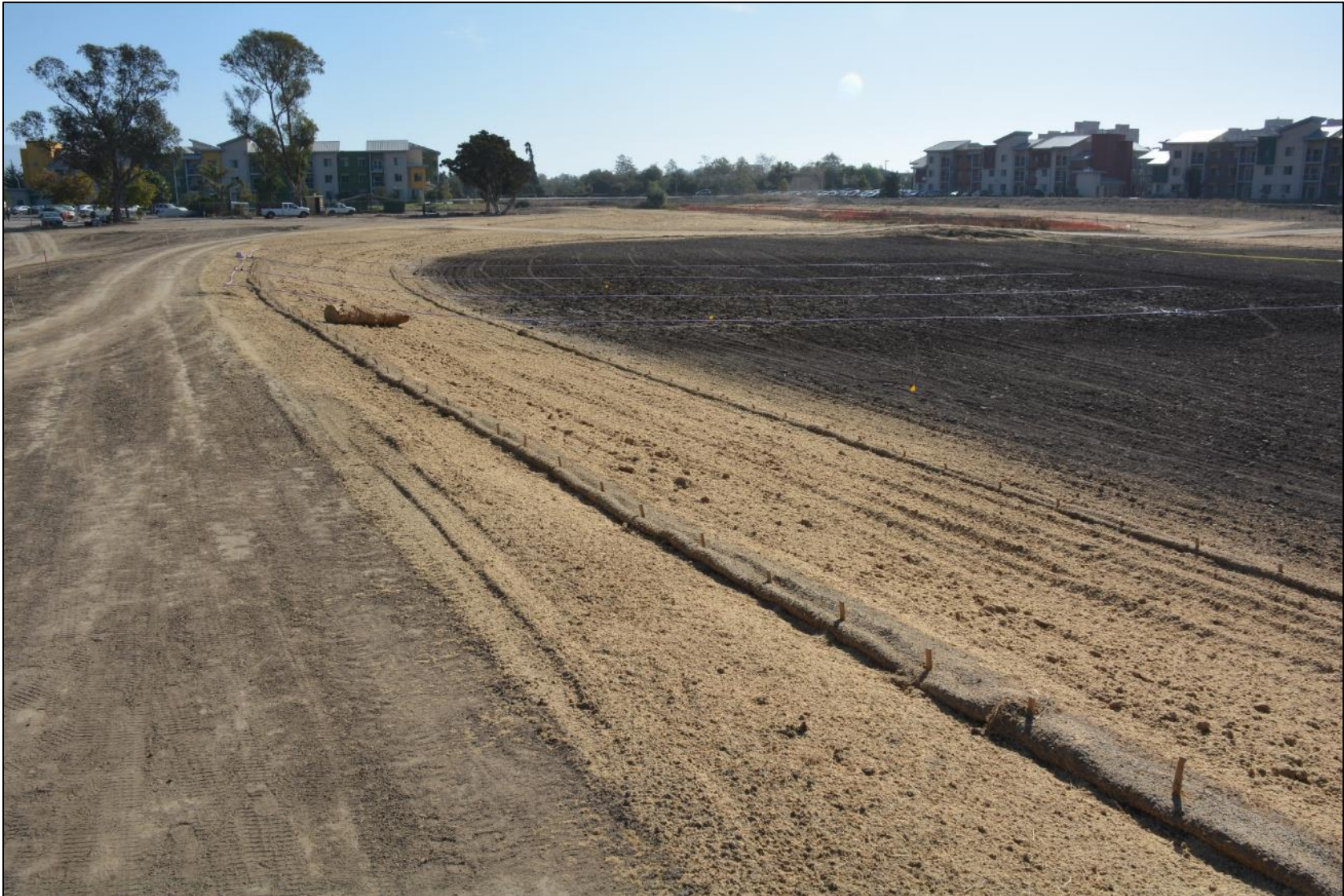
Baseline photo – post-grading, October 10, 2017.
