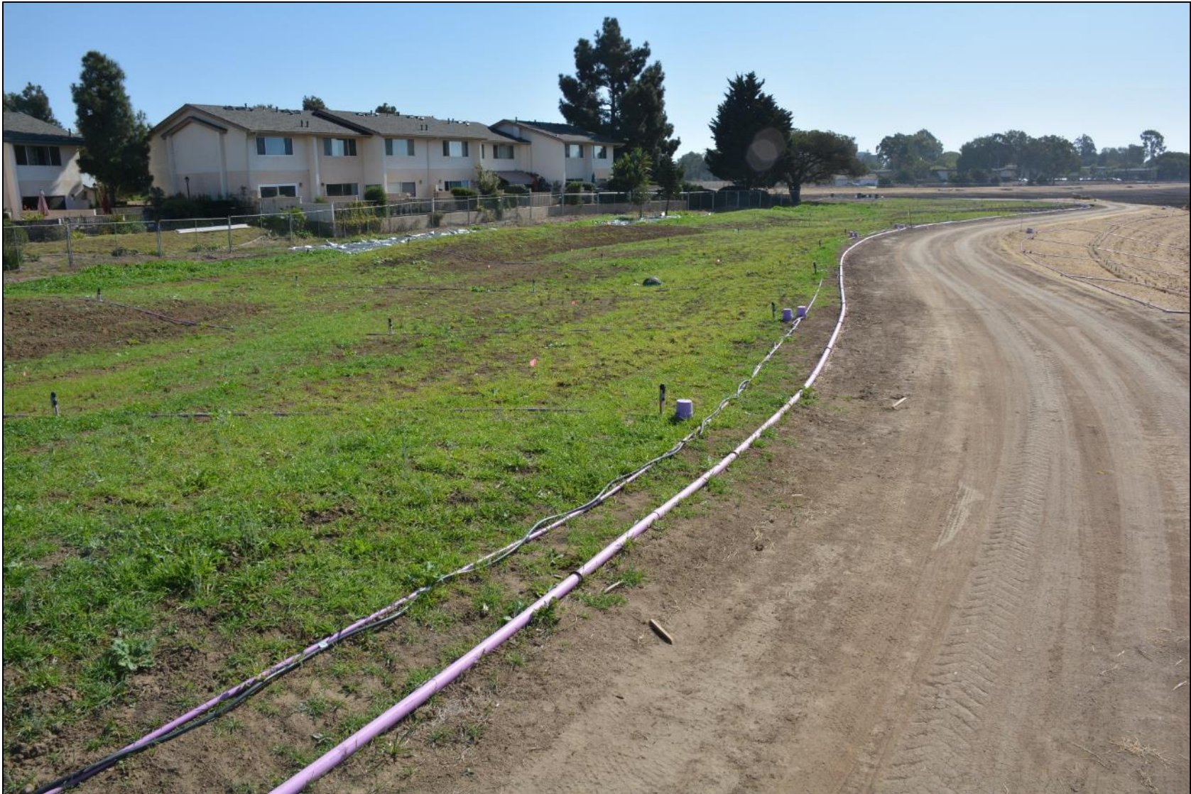
Baseline photo – post-grading, October 10, 2017.
