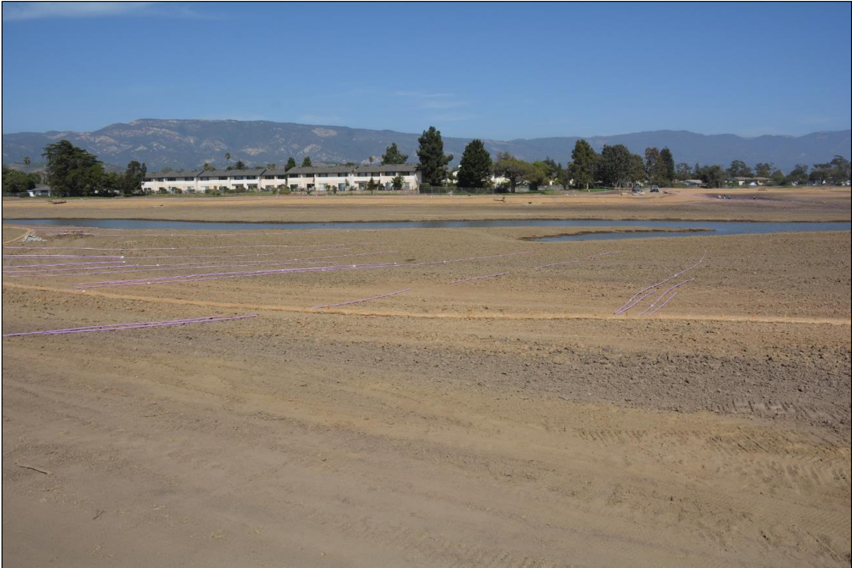
Baseline photo – post-grading, October 10, 2017.
