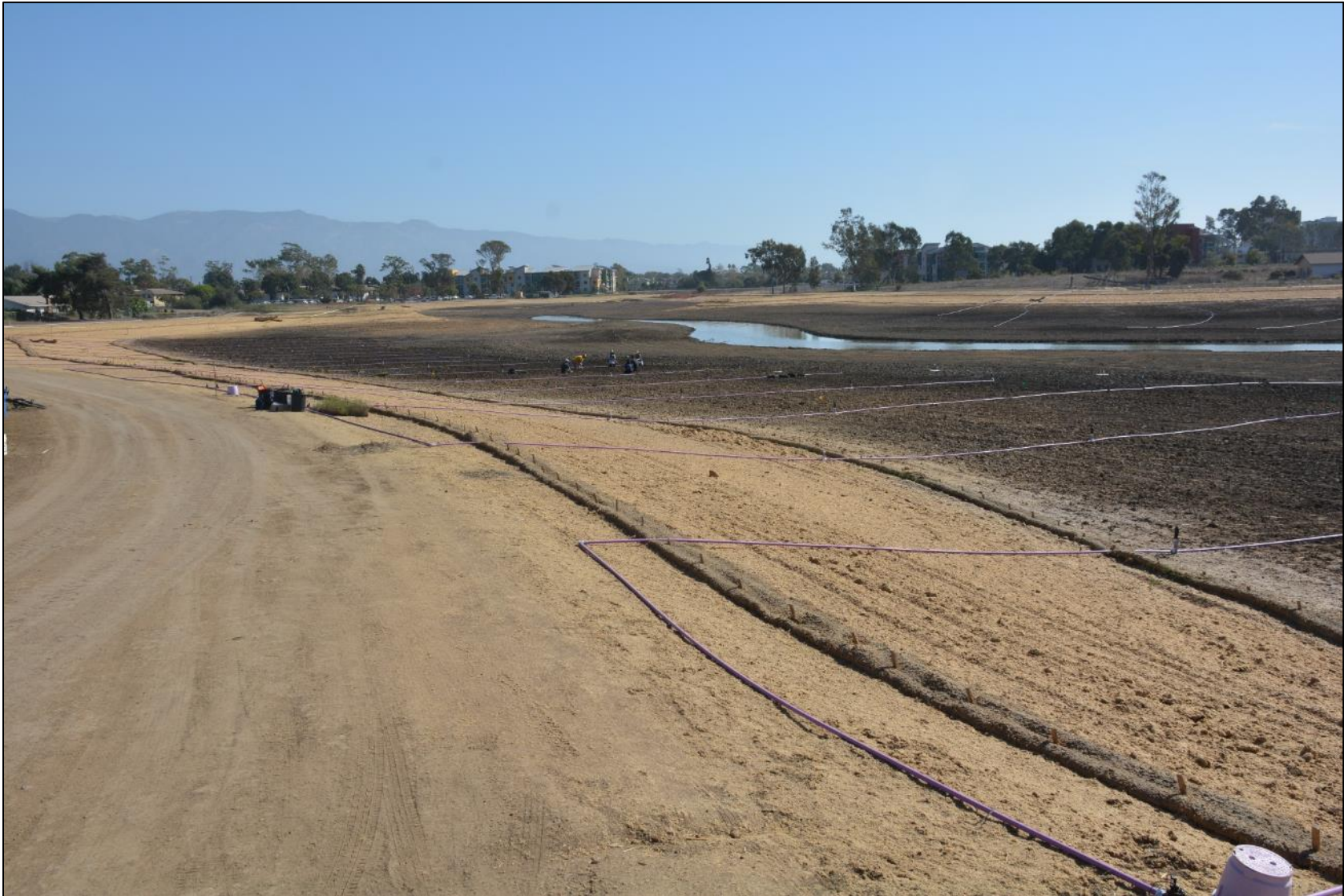
Baseline photo – post-grading, October 10, 2017.
