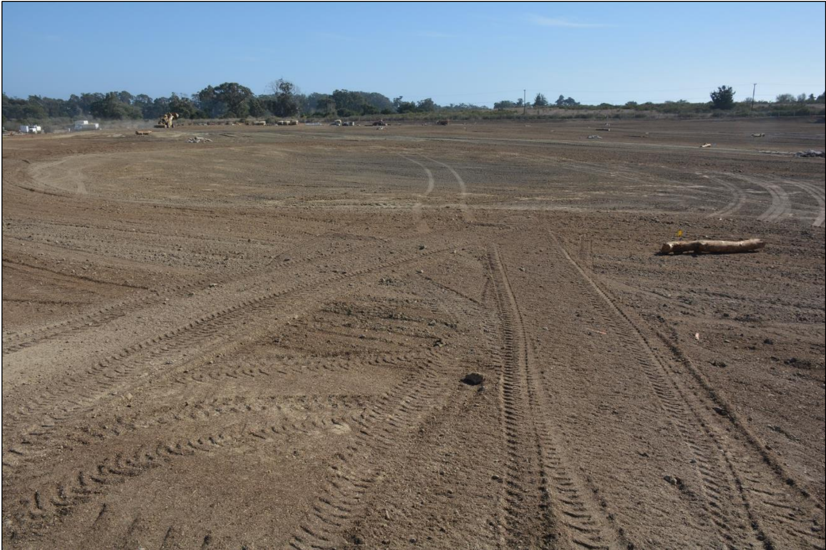
Baseline photo – post-grading, October 10, 2017.
