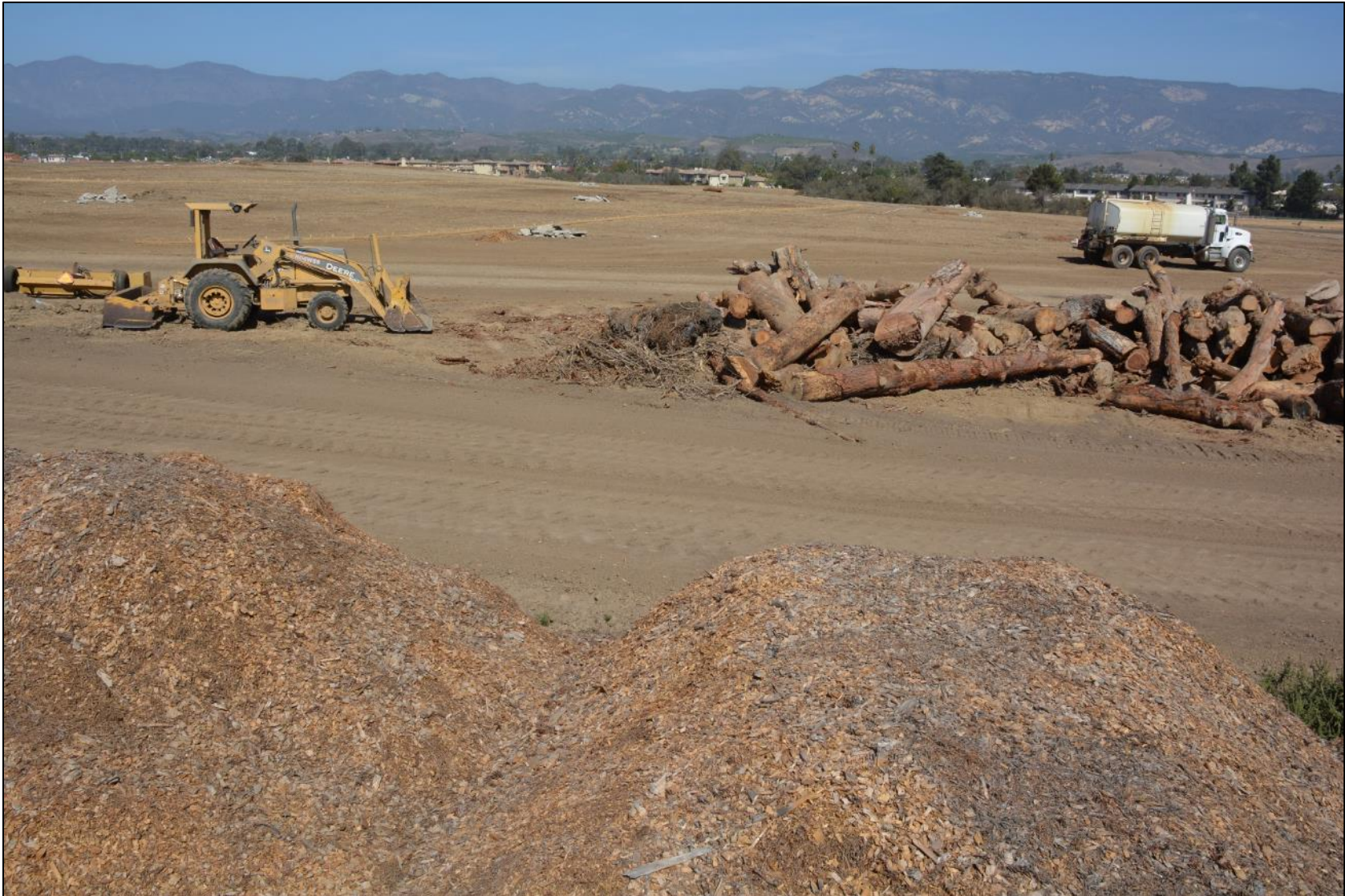
Baseline photo – post-grading, October 10, 2017.
