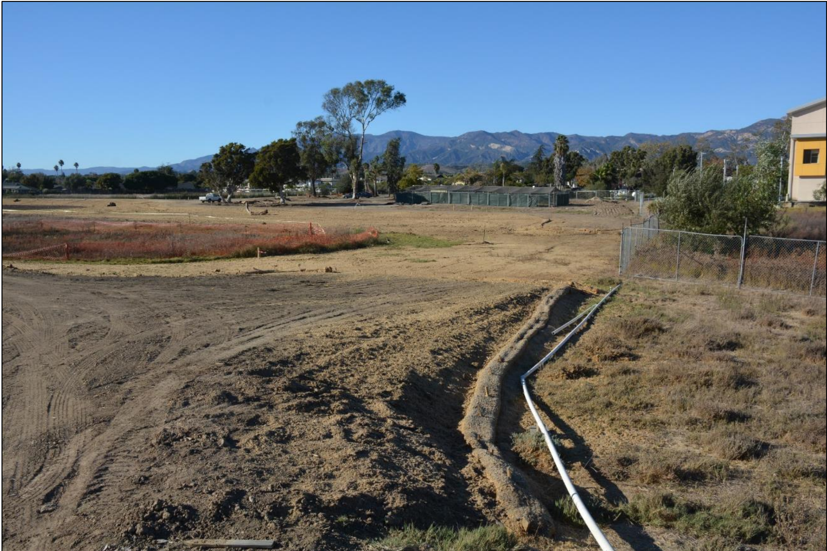
Baseline photo – post-grading, October 24, 2017.
