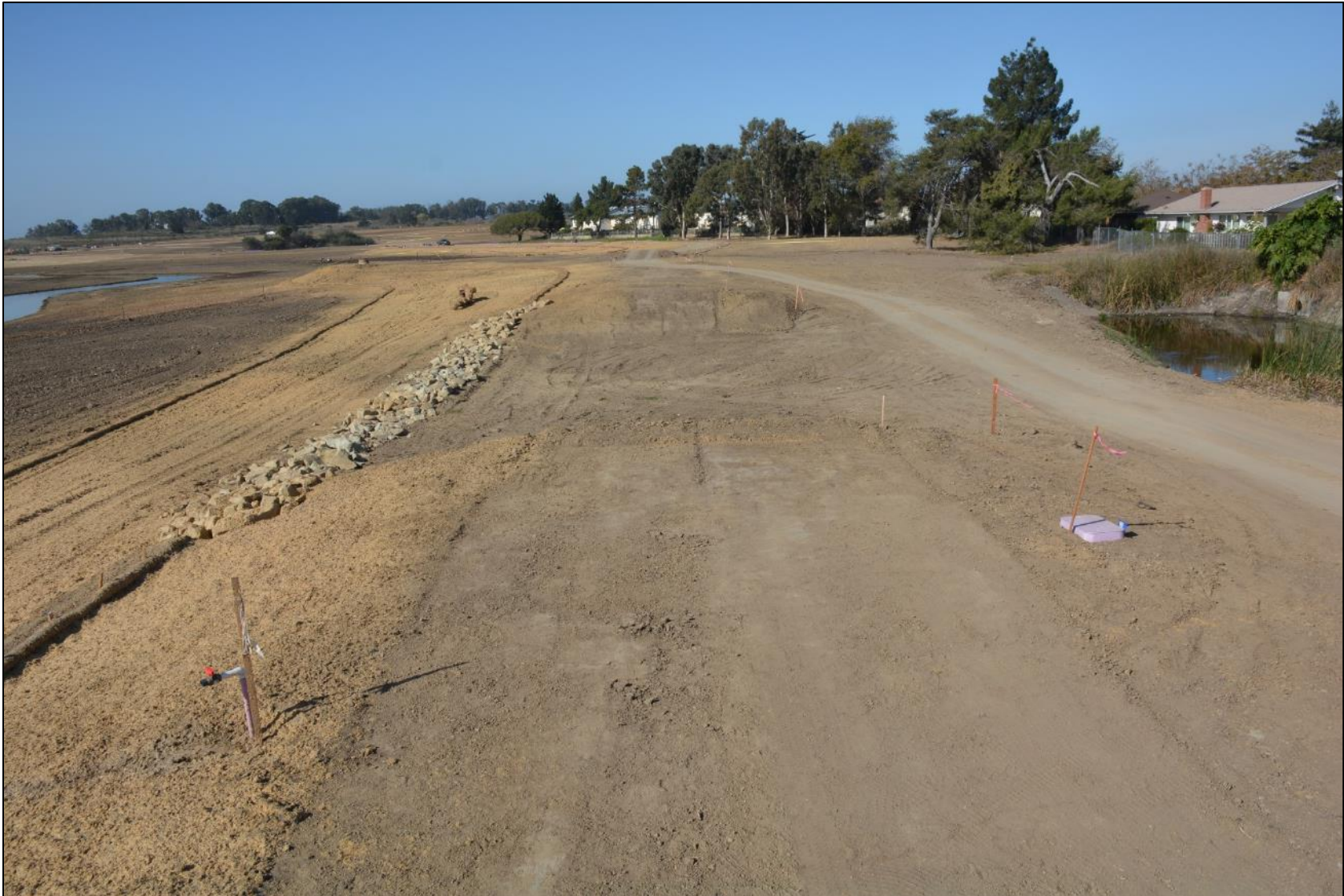
Baseline photo – post-grading, October 10, 2017.
