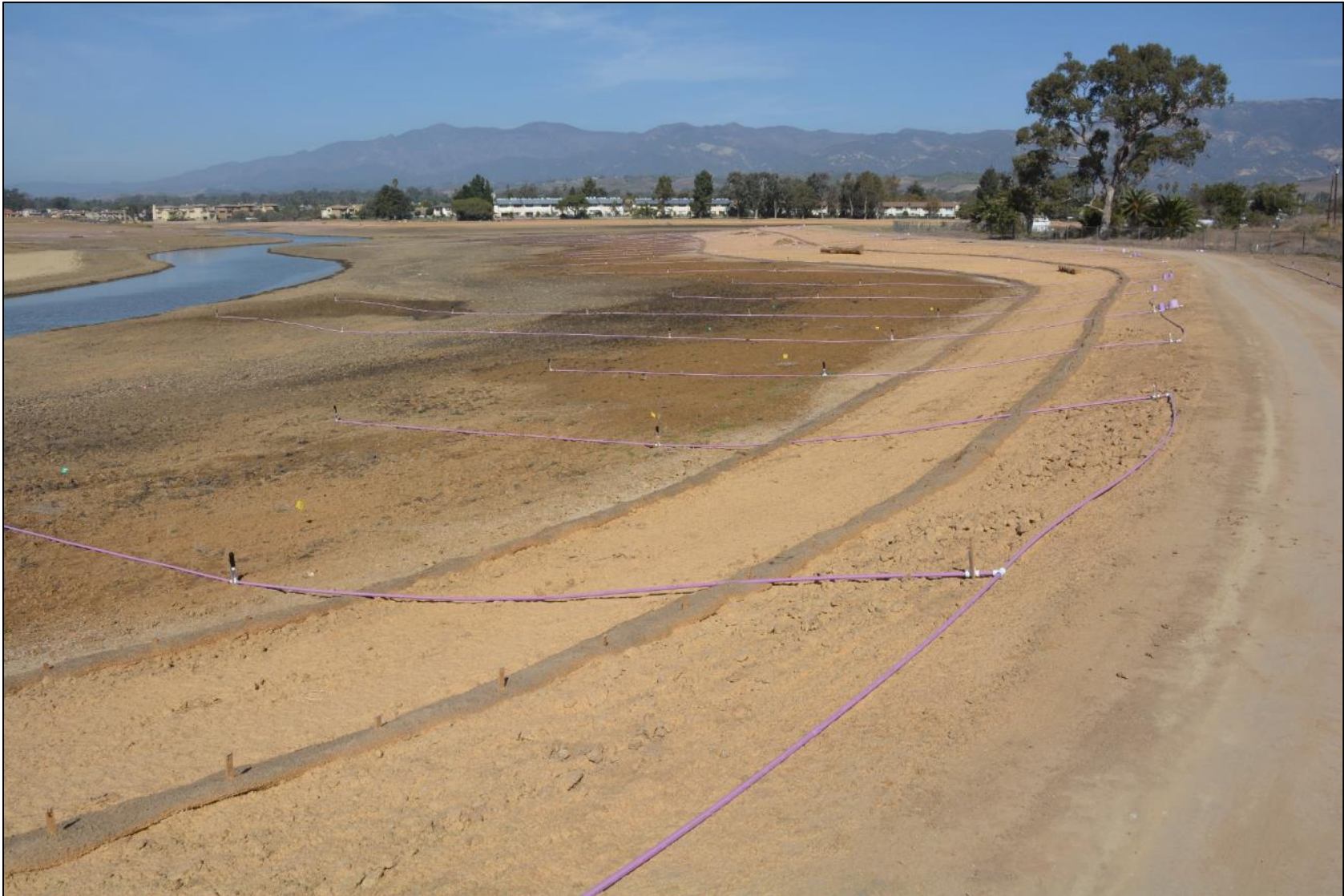
Baseline photo – post-grading, October 10, 2017.
