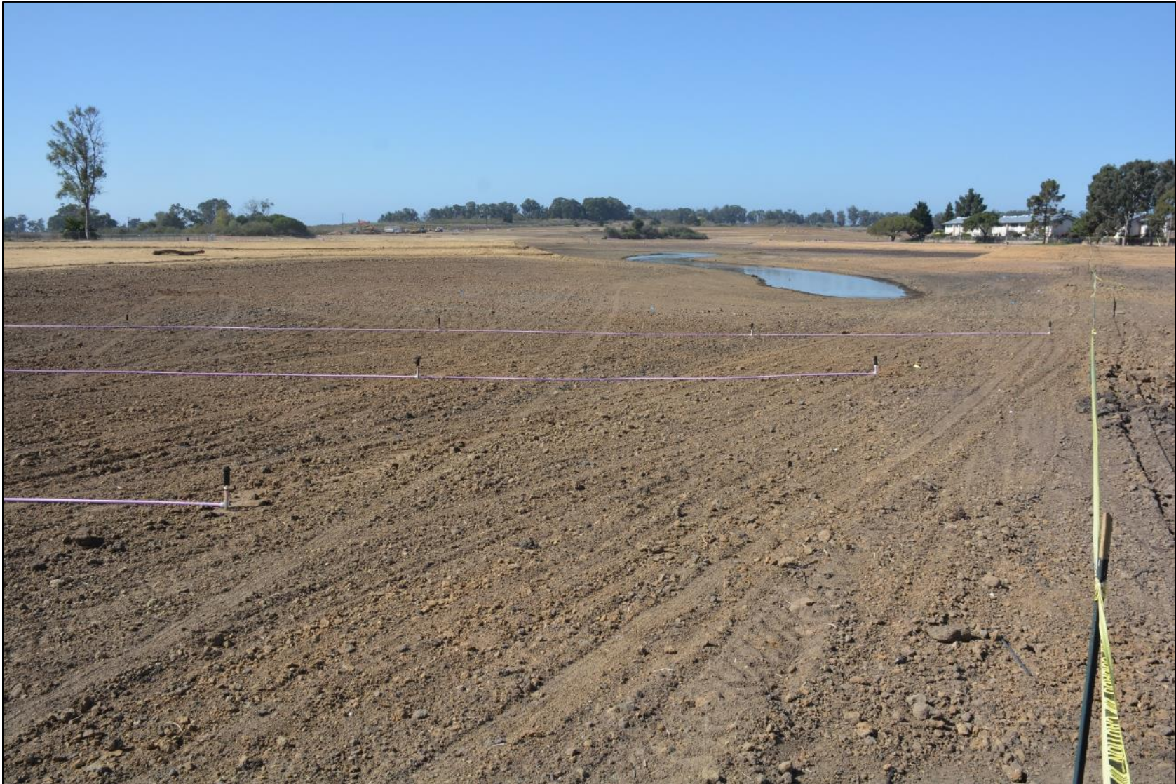
Baseline photo – post-grading, October 10, 2017.
