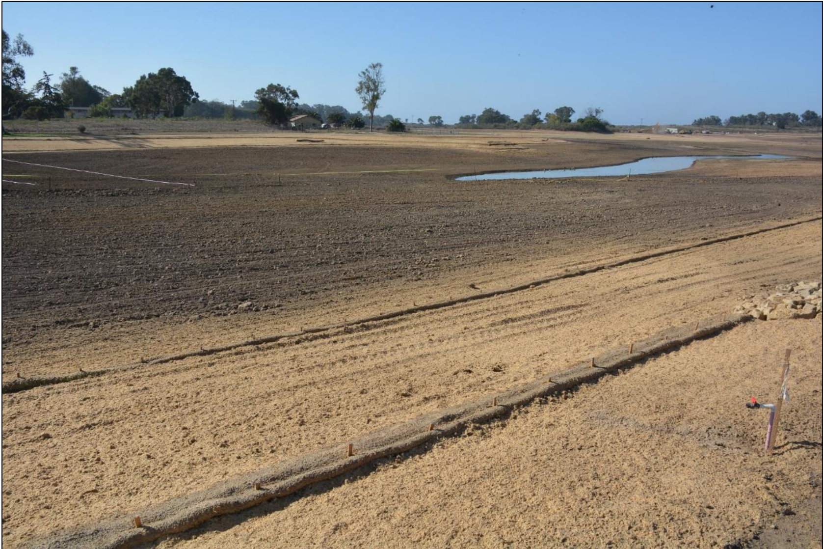
Baseline photo – post-grading, October 10, 2017.
