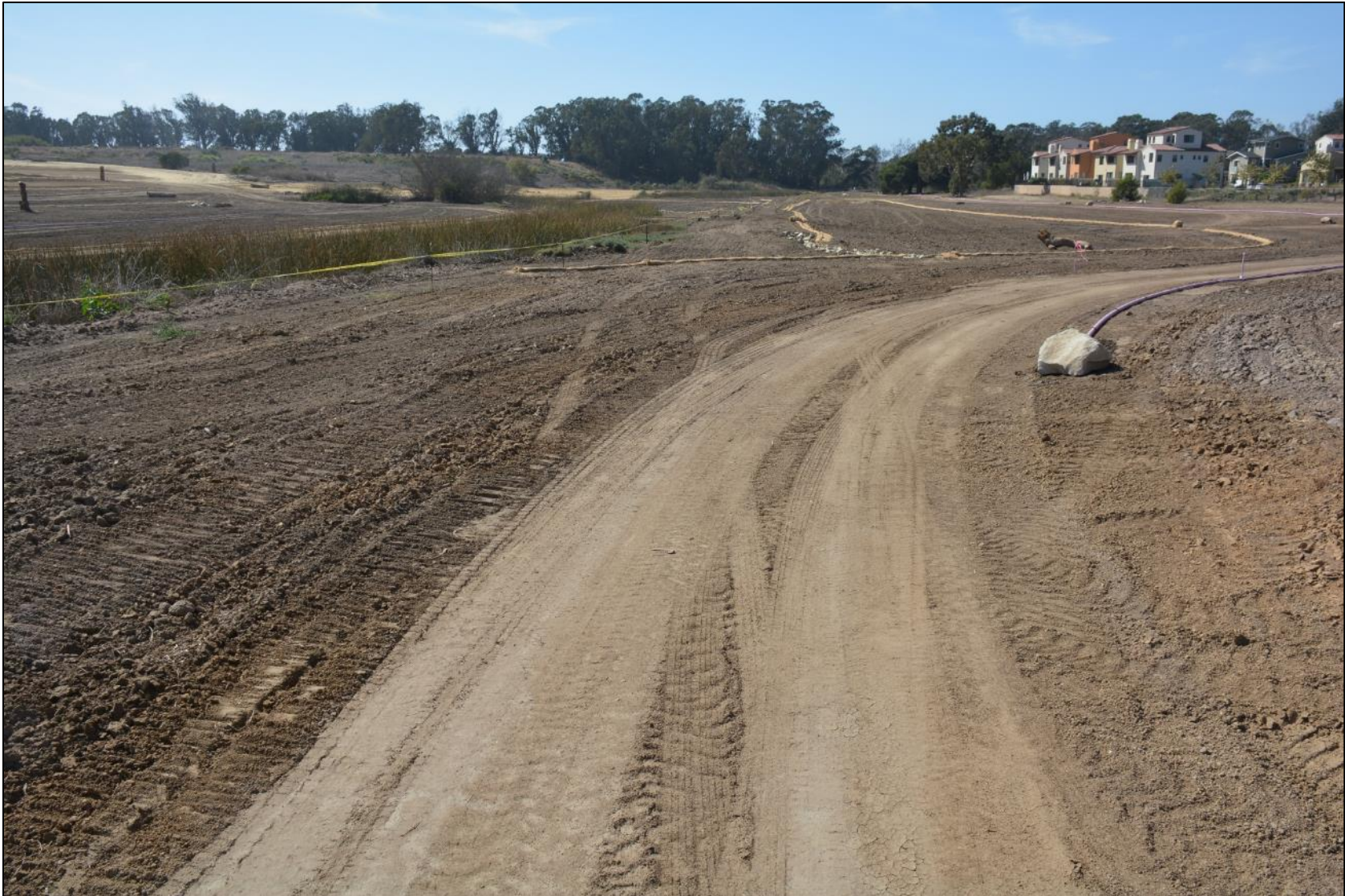
Baseline photo – post-grading, October 10, 2017.
