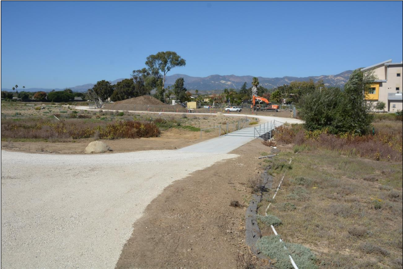
Year 1 photo – October 15, 2018. Note completion of culvert crossing and trail.
