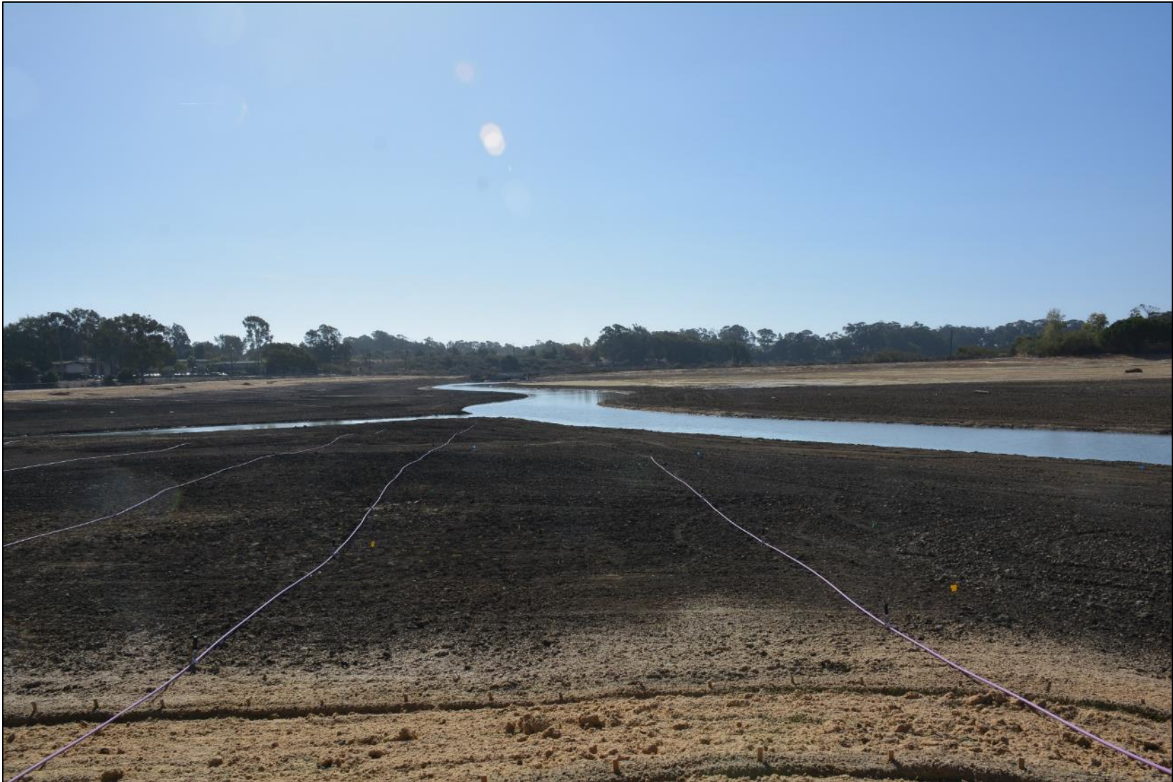
Baseline photo – post-grading, October 10, 2017.
