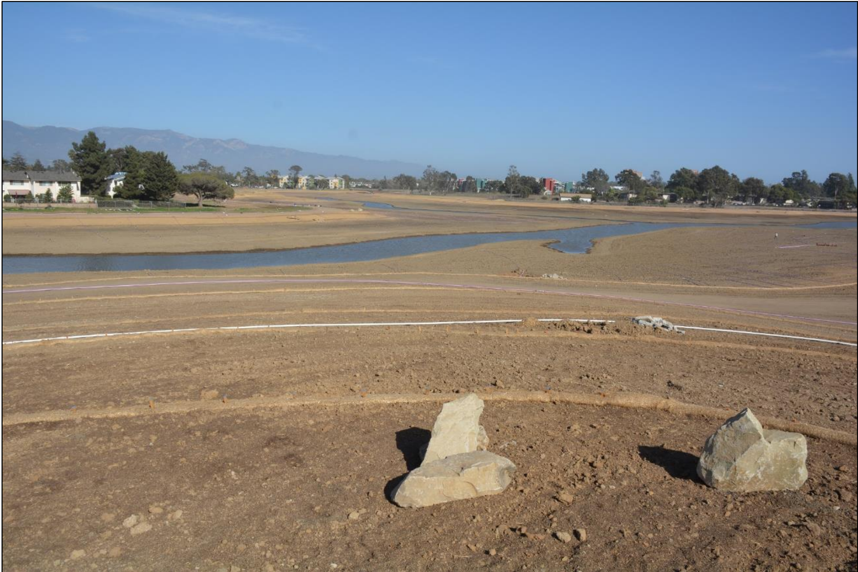
Baseline photo – post-grading, October 10, 2017.
