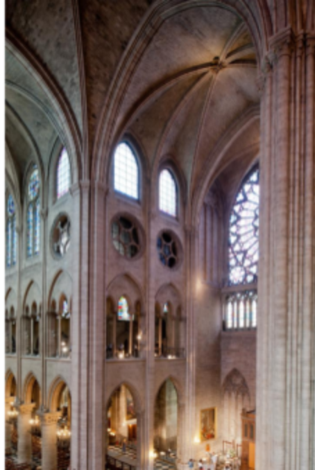
Figure 2.8 Image of four-story elevation. Here, from top to bottom, you can see the clerestory windows, oculus windows, gallery, and arcade of the North Transept.
