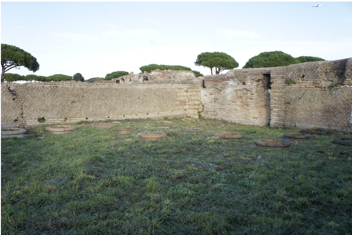
Fig. 3.38. View of Magazzino dei Doli (III.14.3), linked to House of Annius, from south.
