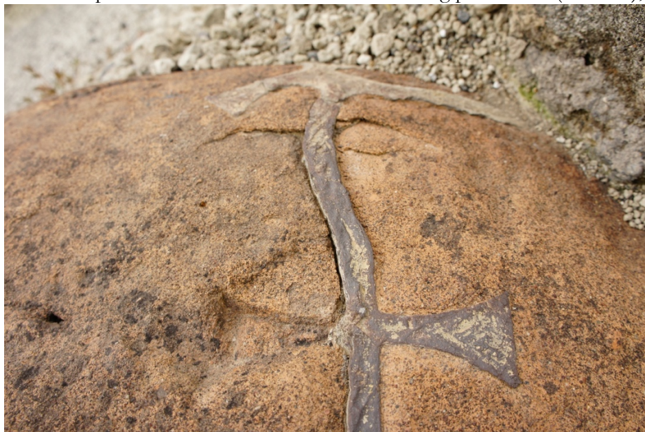
Fig. 4.37. Lead alloy double dovetail tenon, shallow cuttings visible (I.22 n. 3), Pompeii.
