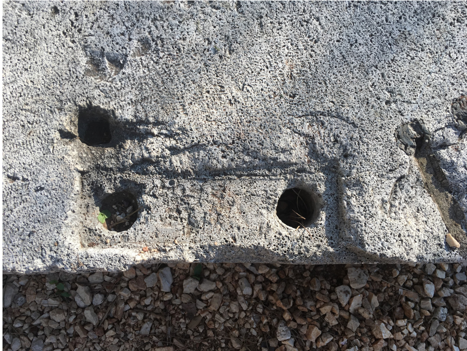
Fig. 4.15. Mortise-and-tenon staple (metal missing) on architectural stone block, in Bass Garden of the American Academy in Rome.
