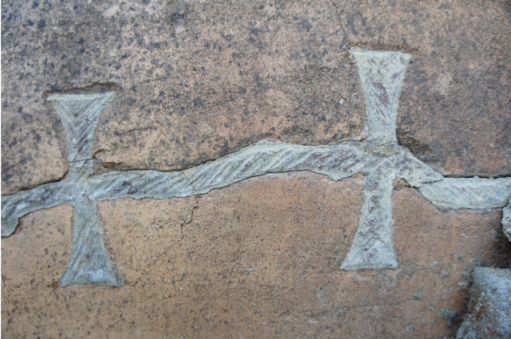
Fig. 4.38. Gouges on surface of lead (alloy?) double dovetail tenon (I.22 n. 3), Pompeii.
