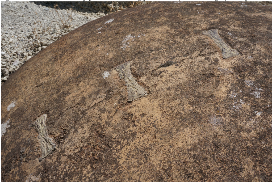
Fig. 4.33. Three double dovetails and clay smeared over horizontal crack that emerged during production phase (I.22 n. 3), Pompeii.
