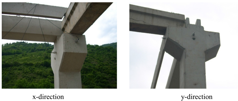
Fig. 16. The accelerometer connections for the precast production facility.
