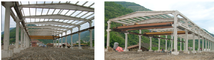
Fig. 15. Some views from precast production facility.
