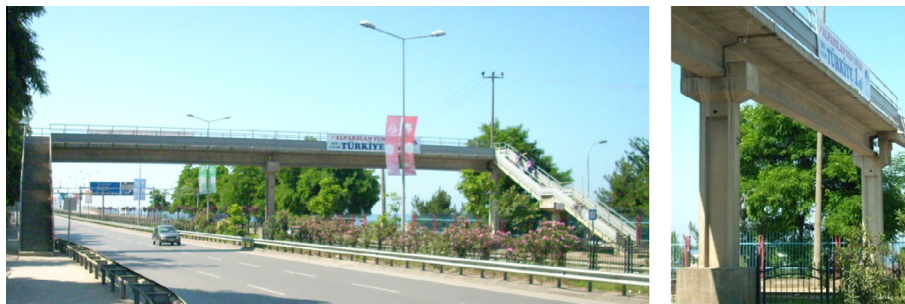
Fig. 2. Some views from C-1 overpass.
